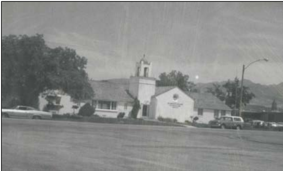
Figure 6. South elevation of the Mexican Branch meetinghouse, ca. 1970 (courtesy of the Church History Department, Church of Jesus Christ of Latter-day Saints).
