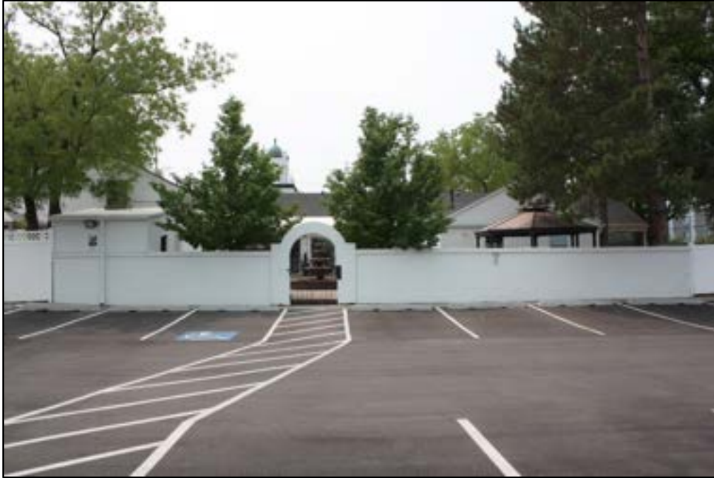
Photo 13 of 54. Overview of the Mexican Branch meetinghouse north elevation. Camera facing south.
