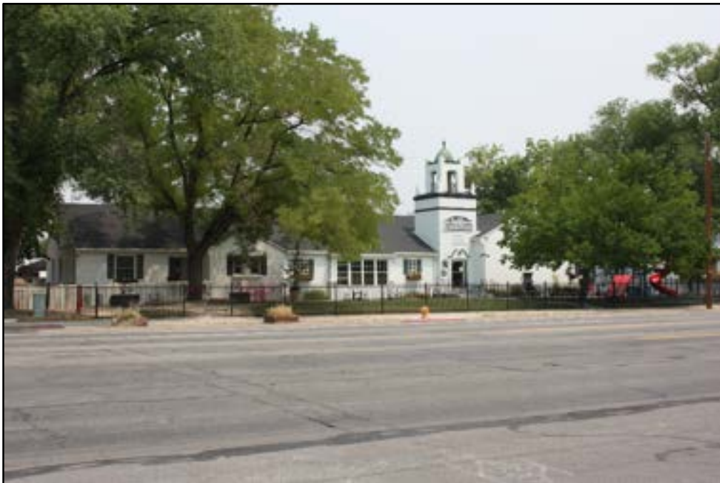
Photo 2 of 54. Overview of the Mexican Branch meetinghouse south (primary) elevation. Camera facing northeast.
