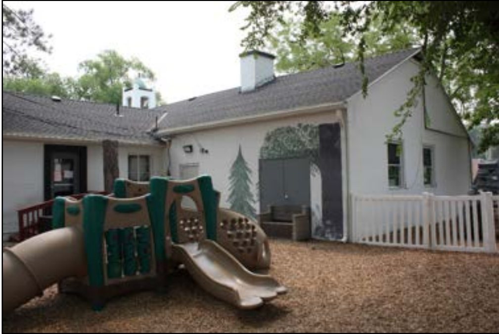
Photo 19 of 54. North and west elevations of the west addition to the Mexican Branch meetinghouse. Camera facing southeast.
