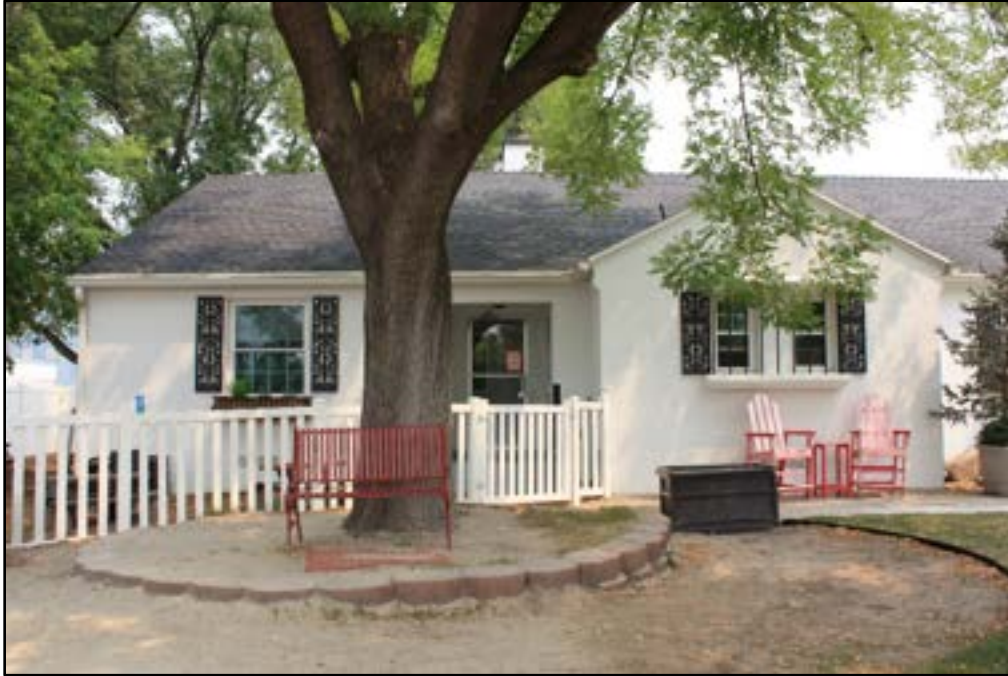
Photo 3 of 54. West addition (left) and the original Mexican Branch meetinghouse, Bays A, B, and C of the south elevation. Camera facing north.
