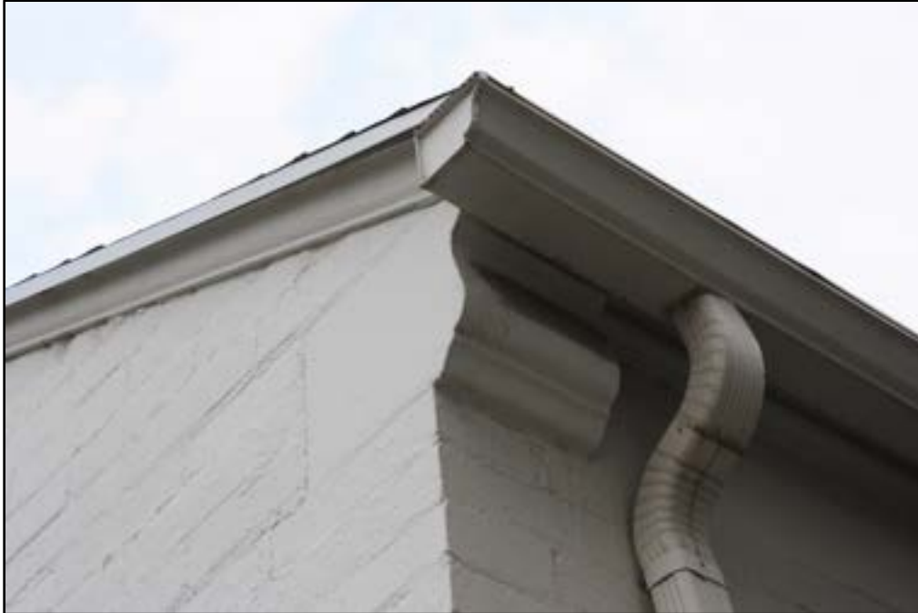
Photo 9 of 54. Detail of curvilinear quoin bracket at the southeast corner of the east wing. Camera facing northwest.
