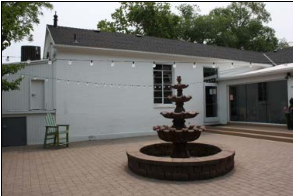
Photo 14 of 54. West elevation of the chapel in the east wing of the Mexican Branch meetinghouse (left) and the north elevation of the recreation/cultural hall (right). Camera facing east.
