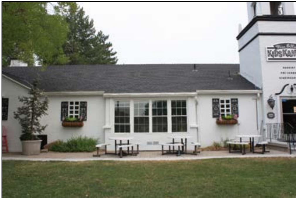
Photo 6 of 54. Original Mexican Branch meetinghouse, Bays D, E, and D of the south elevation. Camera facing north.
