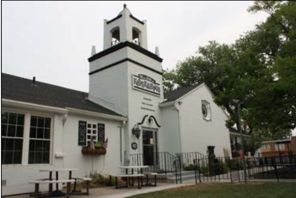
Photo 7 of 54. Original Mexican Branch meetinghouse entrance, Bays F and G of the south elevation. Camera facing northeast.
