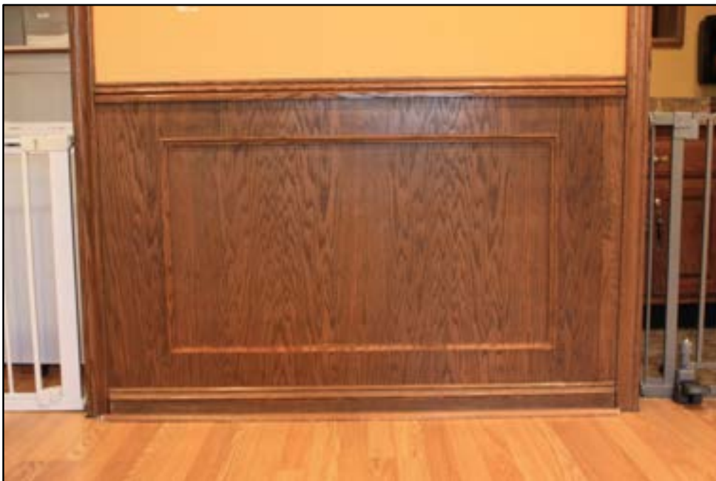
Photo 30 of 54. Detail of original wood wainscoting in the east addition of the Mexican Branch meetinghouse.
