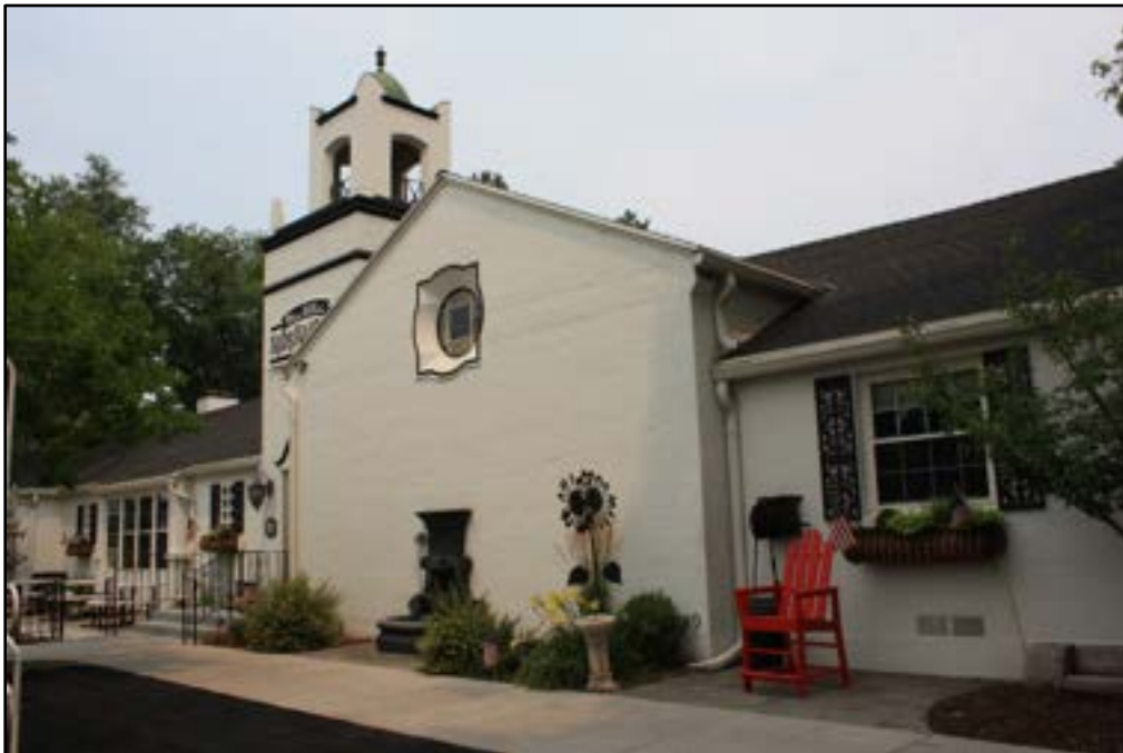
Photo 8 of 54. South end of the chapel in the original Mexican Branch meetinghouse, Bays F and G of the south elevation. Camera facing northwest.
