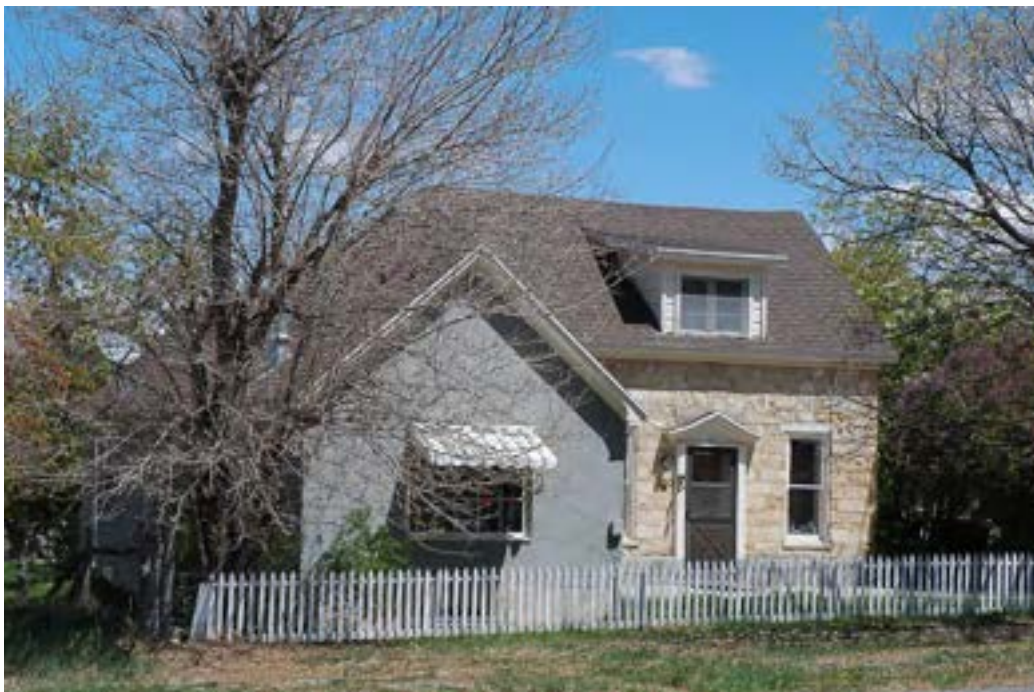
Photograph 50 Stone house with in-period additions at 112 W 200 N. Camera facing north.
