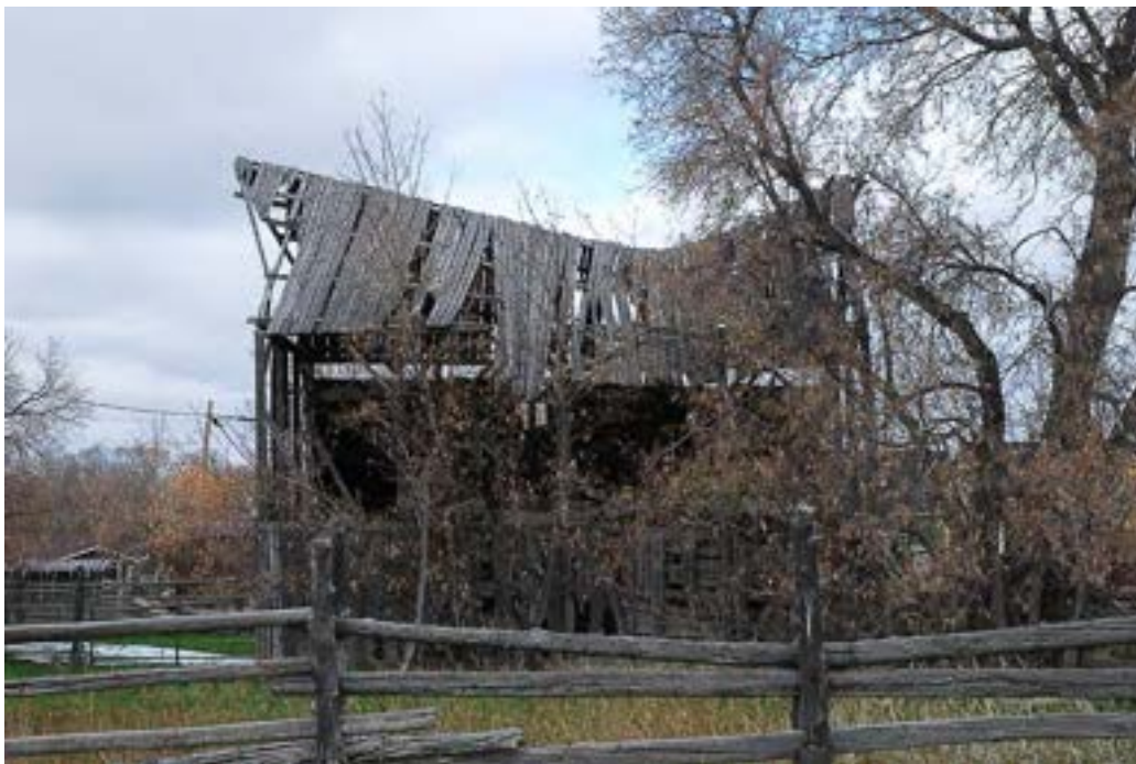
Photograph 14 Barn at 94 E. 400 South. Camera facing north.
