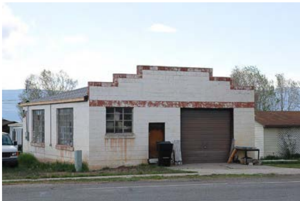
Photograph 46 Concrete block service bay building at 407 N. Main Street. Camera facing west.
