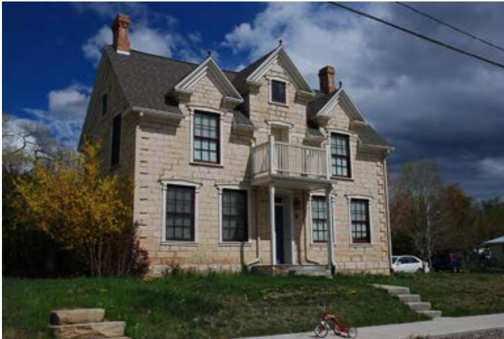
Photograph 17 Stone house at 19 E. 100 North. Camera facing southeast.
