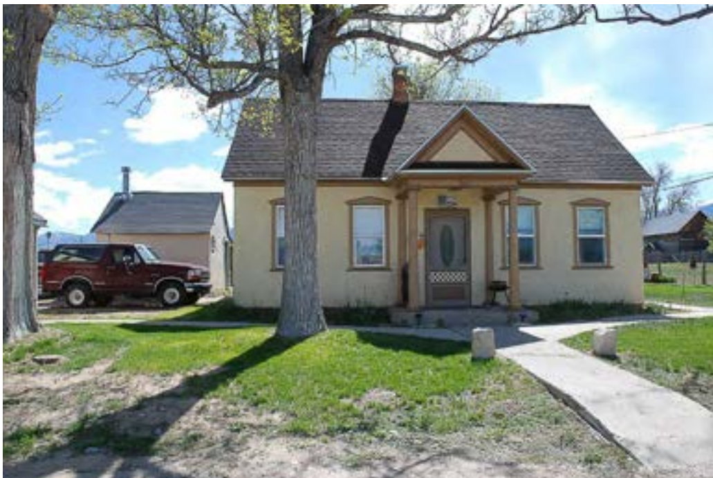
Photograph 18 Stucco-covered house at 560 N. 200 East, summer kitchen on left. Camera facing east.
