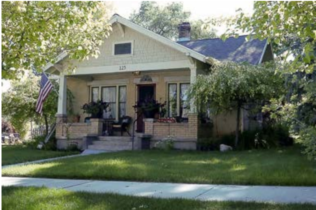
Photograph 51 Brick bungalow at 125 S. Main Street. Camera facing east.
