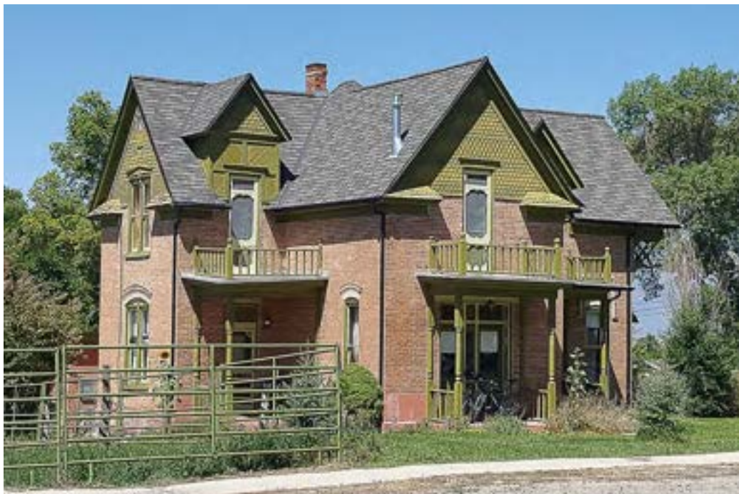
Photograph 28 Brick house at 216 S. Main Street. Camera facing northwest.
