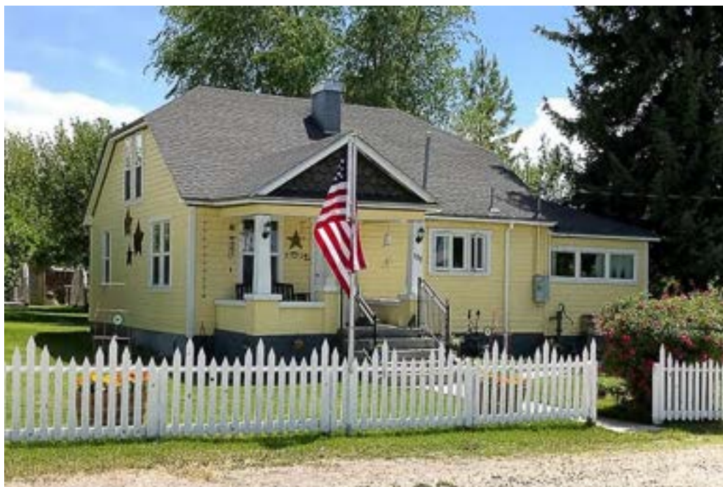
Photograph 52 Clipped-gable period revival frame cottage at 190 E. 500 North. Camera facing south.
