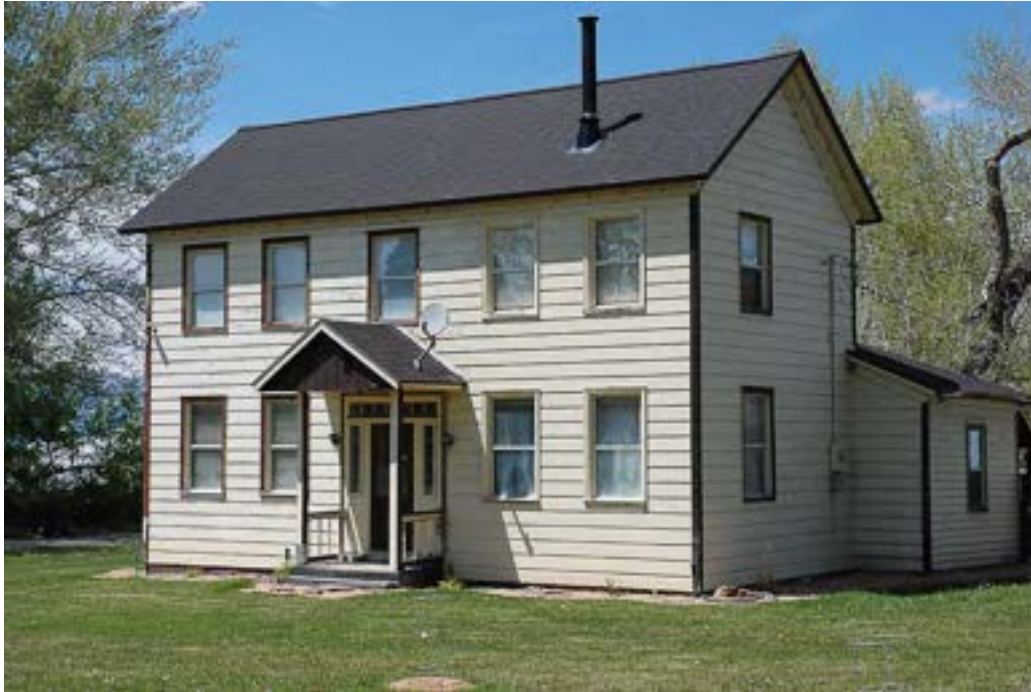
Photograph 23 Frame house at 297 S. 100 West. Camera facing northwest.
