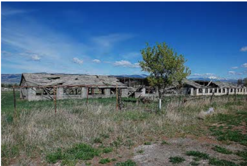
Photograph 48 Commercial coop at 405 N. 100 West. Camera facing northwest.
