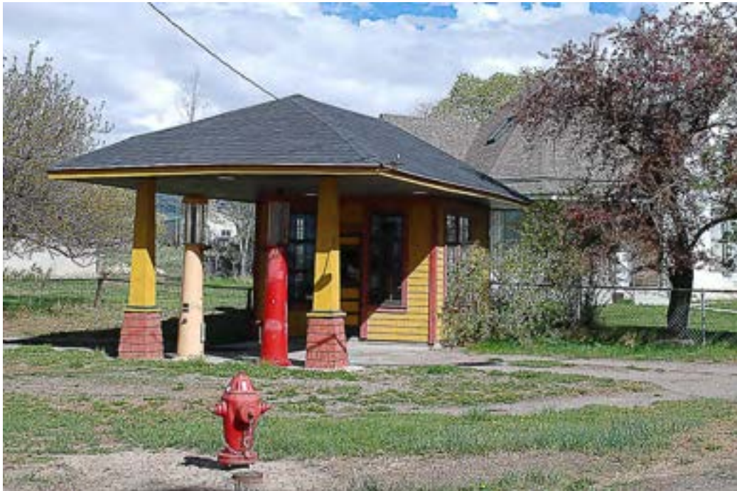
Photograph 43 Early gas station at 498 N. Main Street. Camera facing east.
