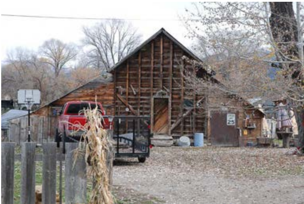
Photograph 24 Inside-out frame barn and granary 297 S. 100 West. Camera facing east.
