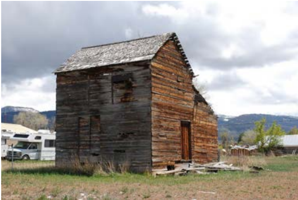
Photograph 49 Grain cleaning shed at 250 E. 100 North. Camera facing northeast.
