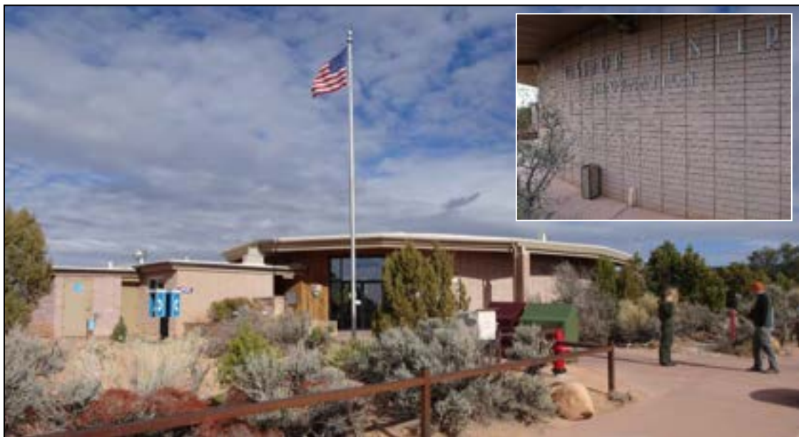
Fig. 4 NABR's Visitor Center, facing northwest, retains its naturalistic landscape softening the original tinted concrete-paved terrace leading into the building past the original flagpole. The recent disabled-access restroom addition is at far left. The land-line telephone stand (blue baffles at left) is a reminder of the monument's very remote location. The recent vinyl roof is barely visible. Inset: Mission 66 metal-letter signage on stack-bond blocks along the wrap-around porch, facing northwest. Both: James Steely, 2018.
