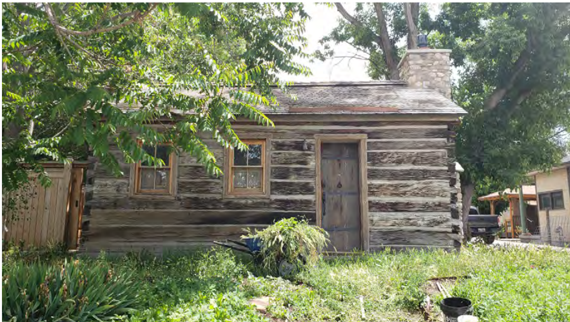
2 of 11. Front/west elevation. Camera facing east.
