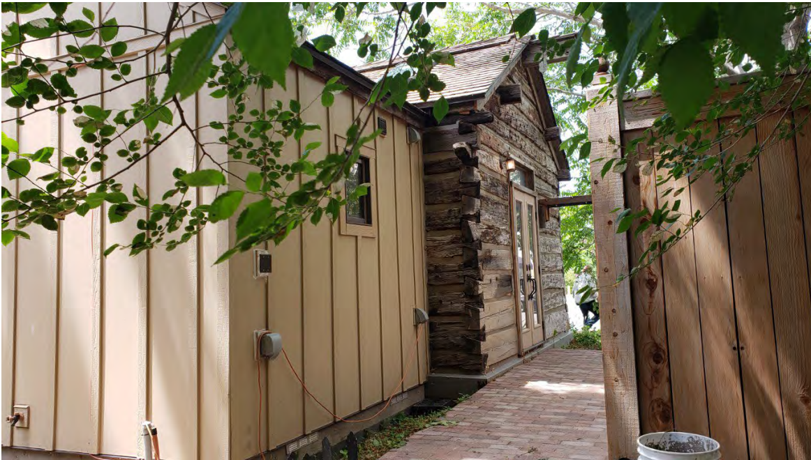
6 of 11. North and east elevations showing patio area. Camera facing southwest.
