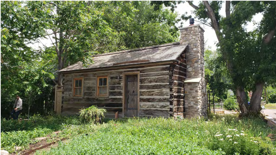
3 of 11. South and west elevations. Camera facing northeast.
