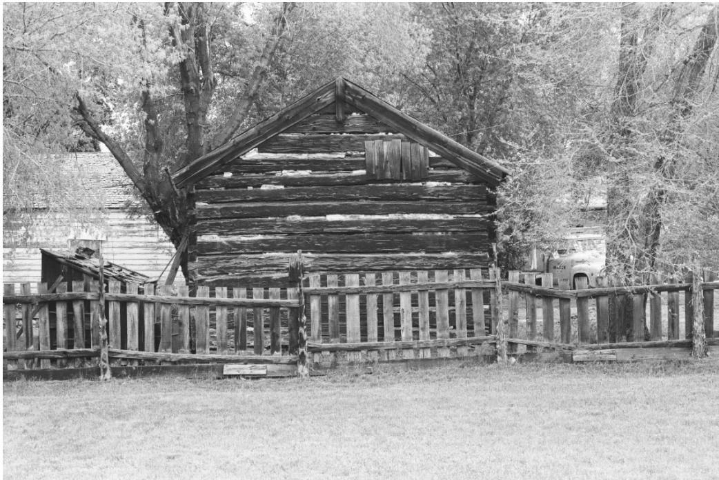
2 of 6. South elevation BEFORE. Camera facing north.
