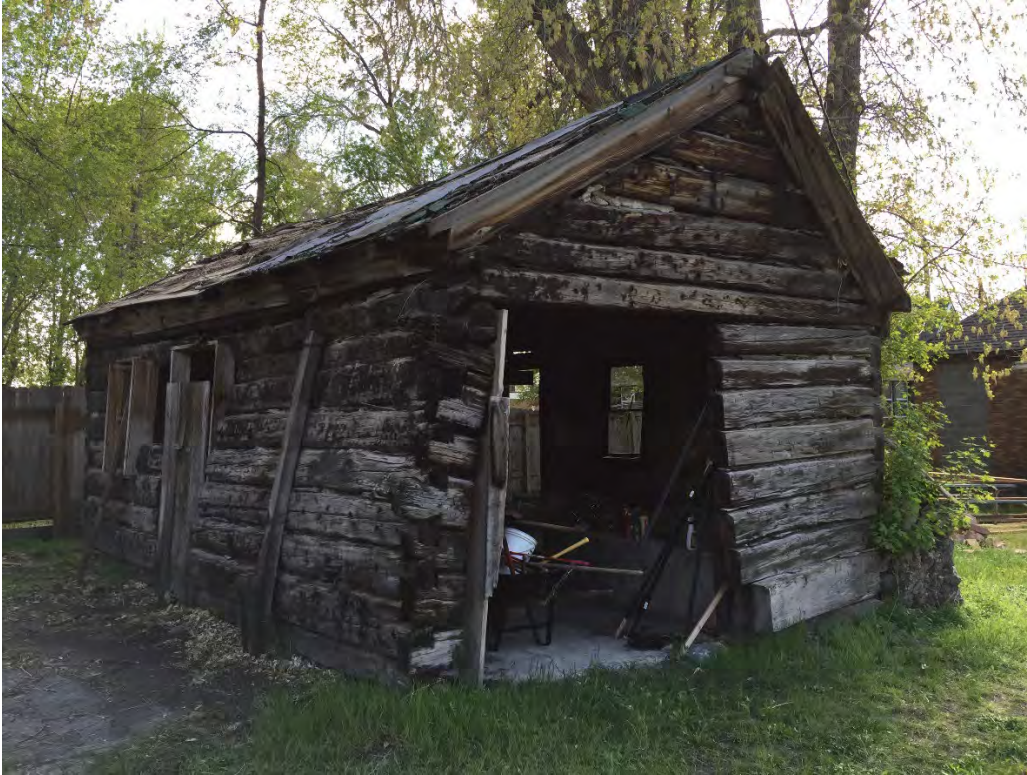
3 of 6. North and east elevations BEFORE. Camera facing Southwest.
