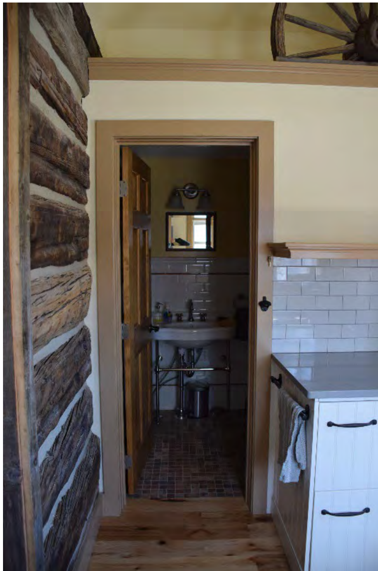
10 of 11. Interior view from inside the addition showing west exterior wall of cabin to the left. Camera facing north.
