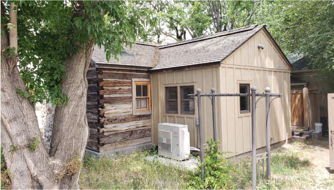
5 of 11. South and east elevations. Camera facing northwest.
