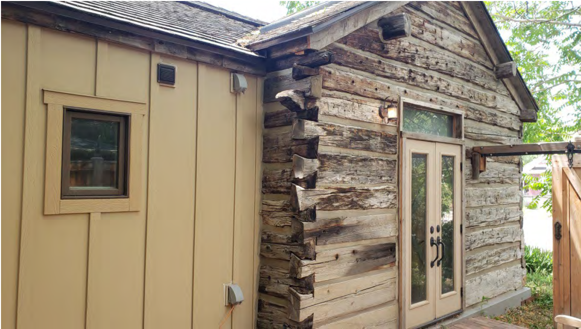
7 of 11. North elevation detail showing addition connection. Camera facing southwest.
