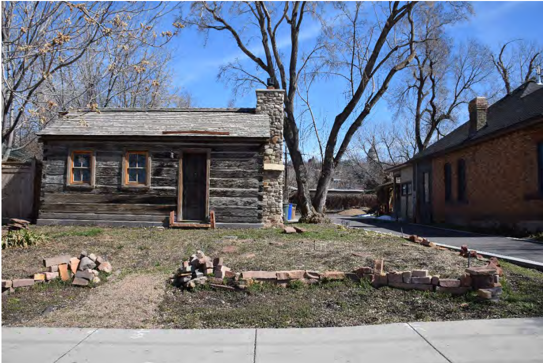
1 of 11. West elevation showing setting. Camera facing east
