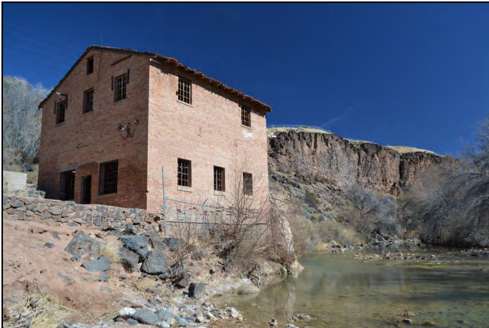
3 of 29. Power Plant on bank of Virgin River. Camera facing east.
