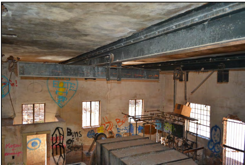
13 of 29. View of ceiling and crane track/support. Camera facing southwest.
