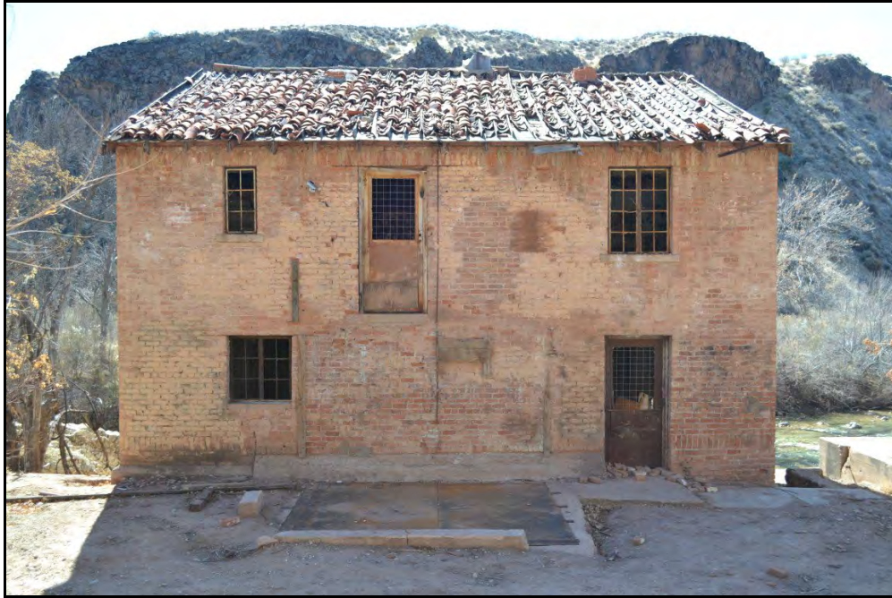
8 of 29. North elevation. Camera facing southwest.
