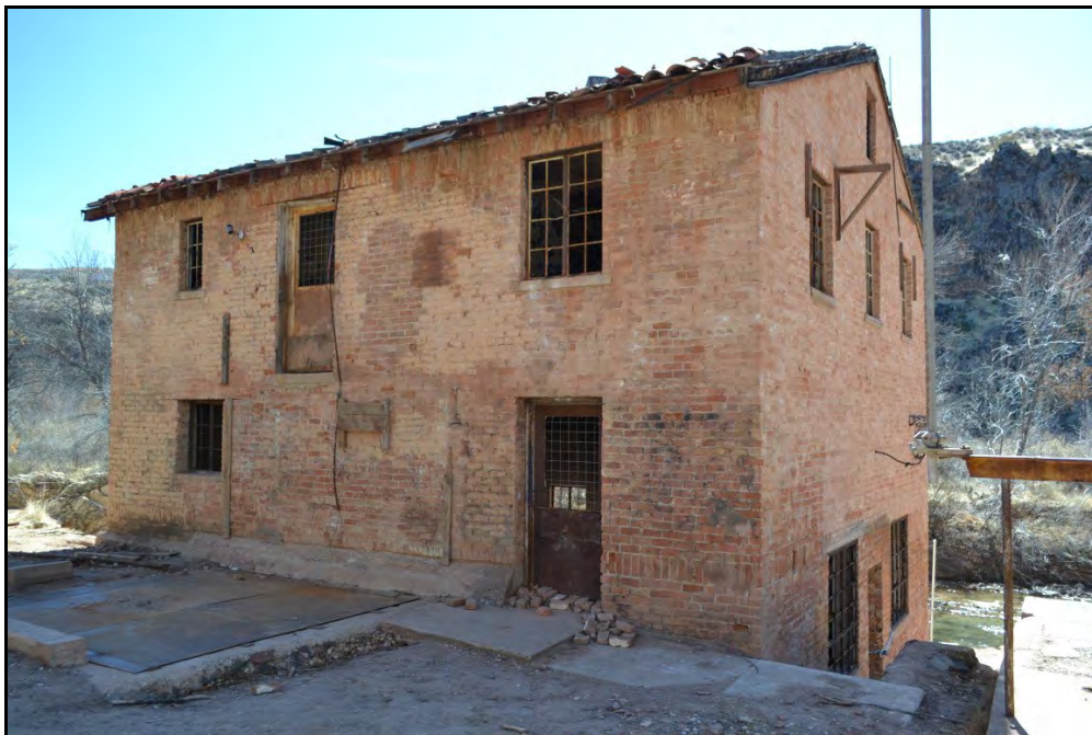
9 of 29. North and west elevation. Camera facing south.
