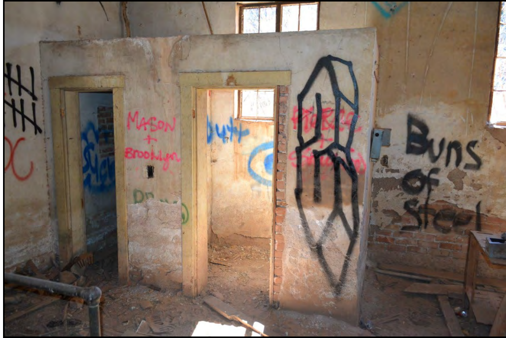
18 of 29. View of small interior rooms, southeast corner. Camera facing southeast.
