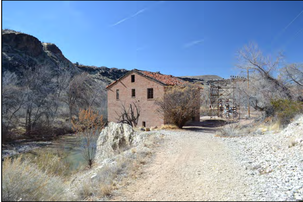
2 of 29. Overview of power plant site from the east. Camera facing west.
