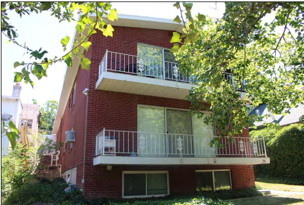
Photograph 7 of 15: Example of Ranch form dwelling; 331 S. 1100 E.; camera facing east
