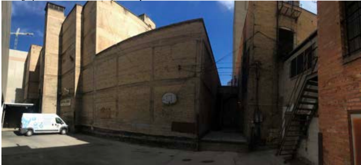
Photograph 3. Exterior, south façade, July 2021. Camera view north.
