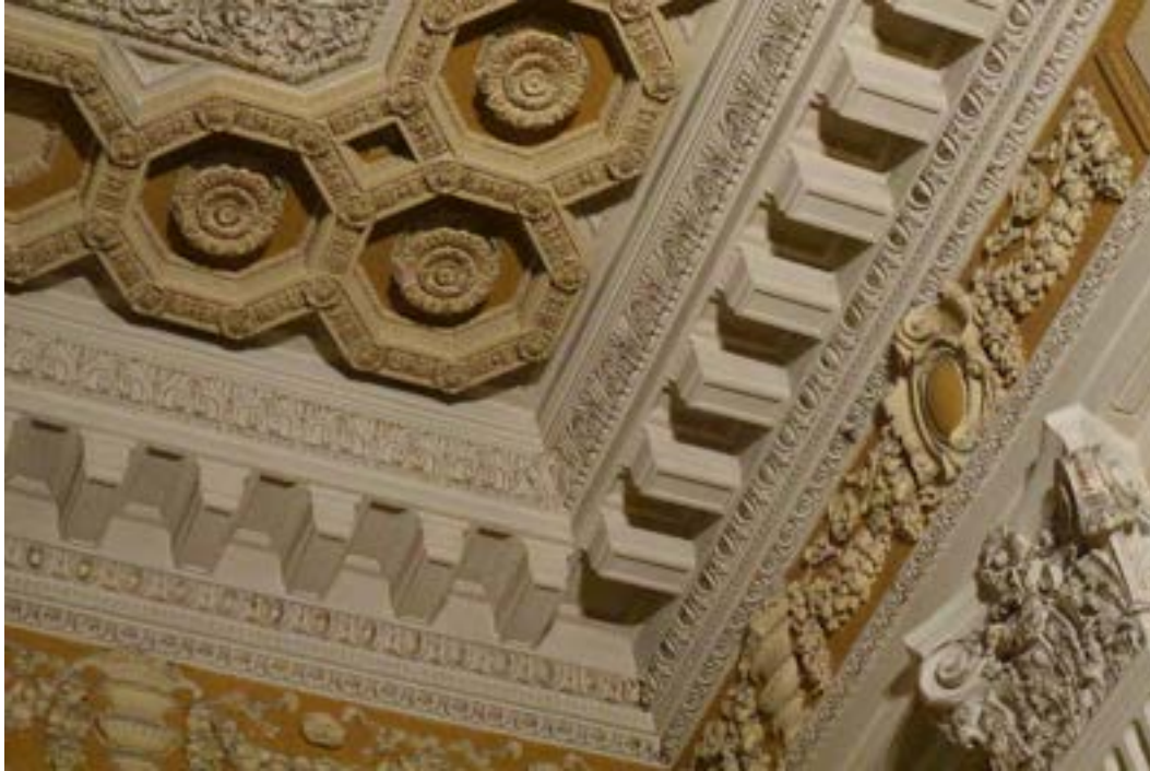
Photograph 11. Interior, Foyer detail, November 2020.
