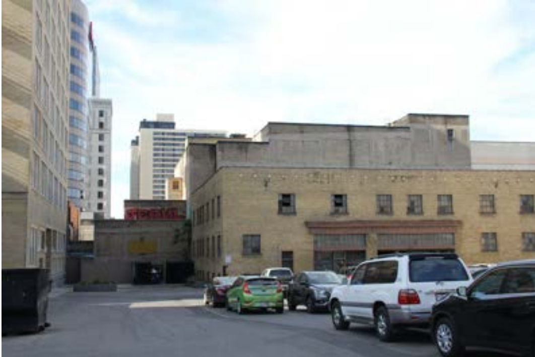
Photograph 5. Exterior, north façade, July 2021. Camera view south.
