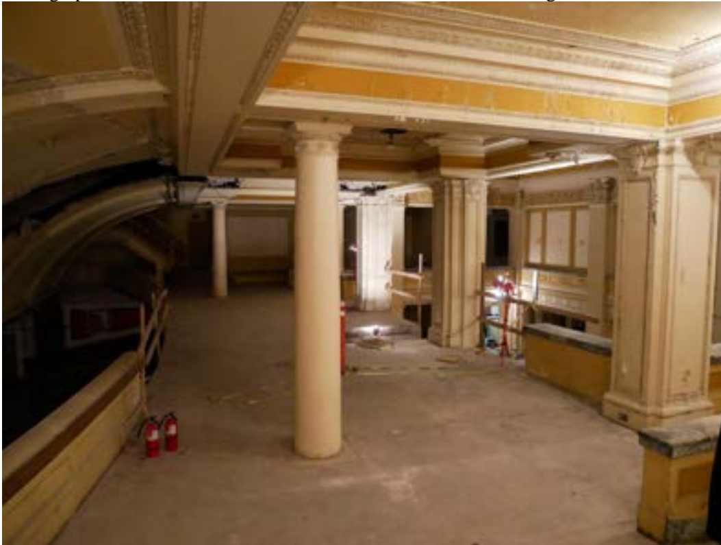
Photograph 12. Interior, Mezzanine, November 2020. Camera facing north.
