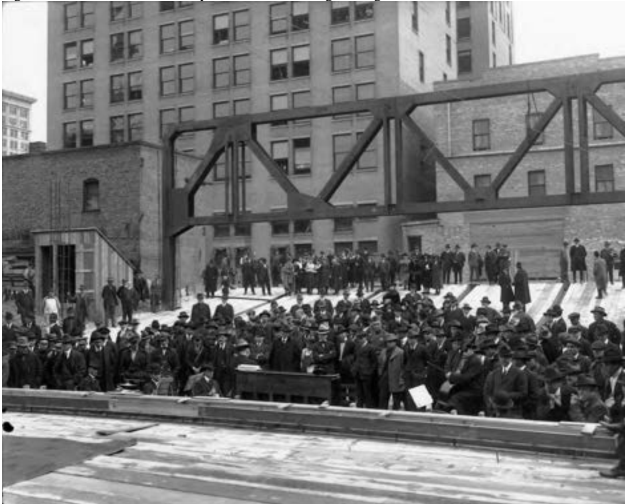
Figure 1. Historic, view of balcony steel beam from stage during construction, 1919.
