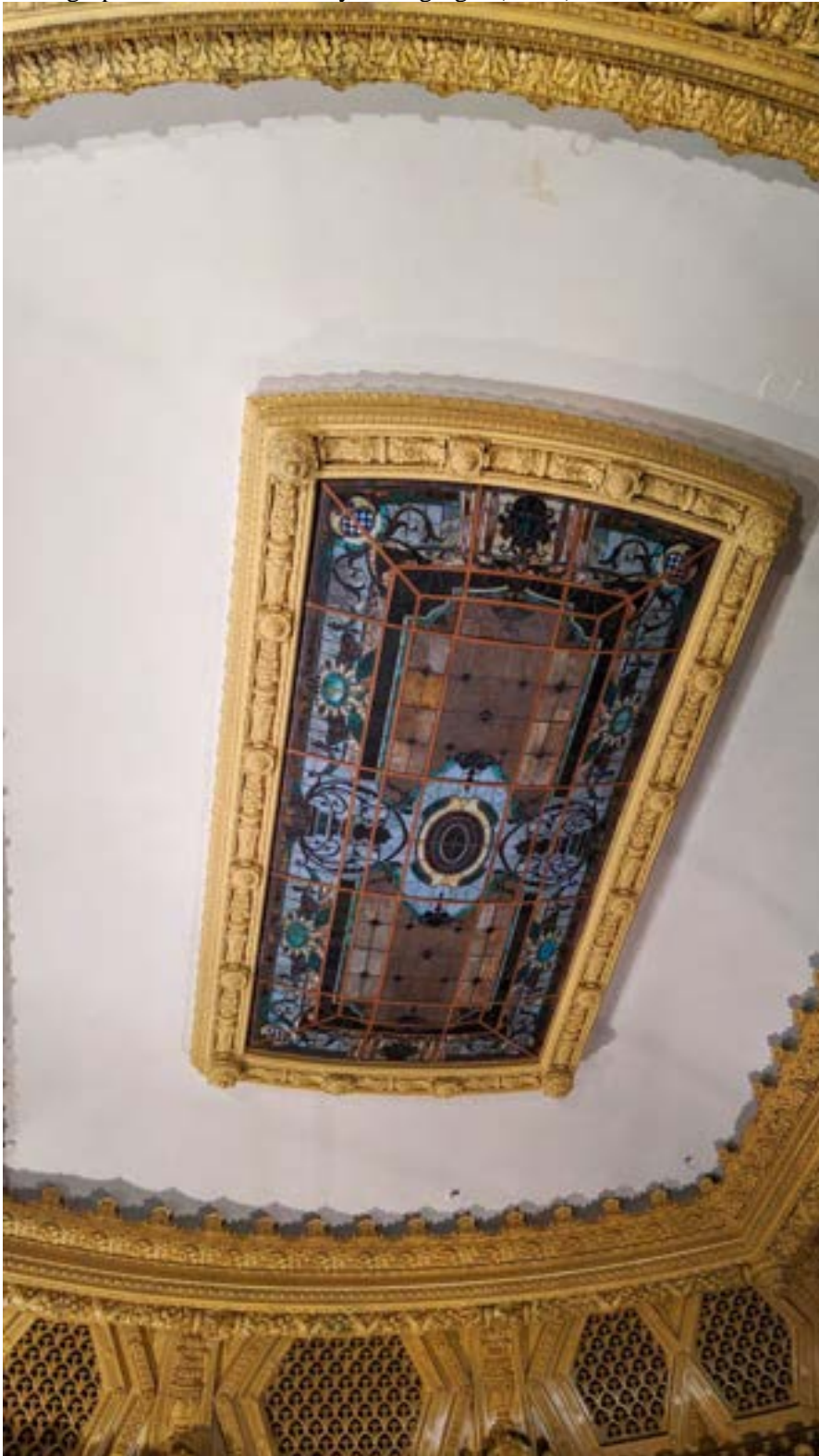
Photograph 15. Interior, Tiffany ceiling light (dome) detail, October 2020.
