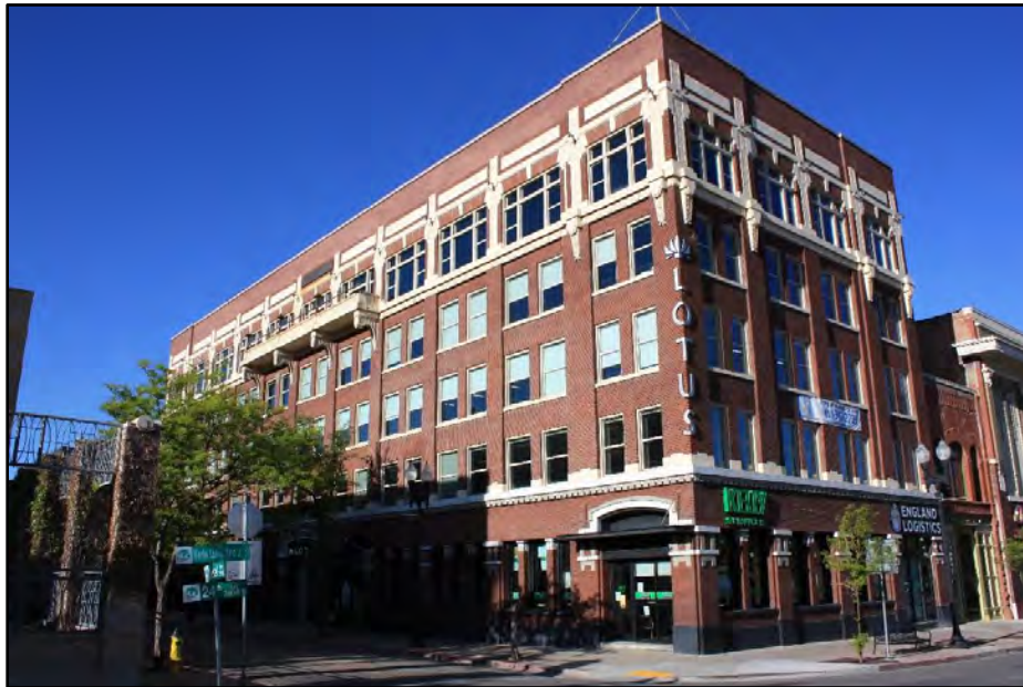
Photo 2. Hudson Building, 2401-2419 Kiesel Avenue.
