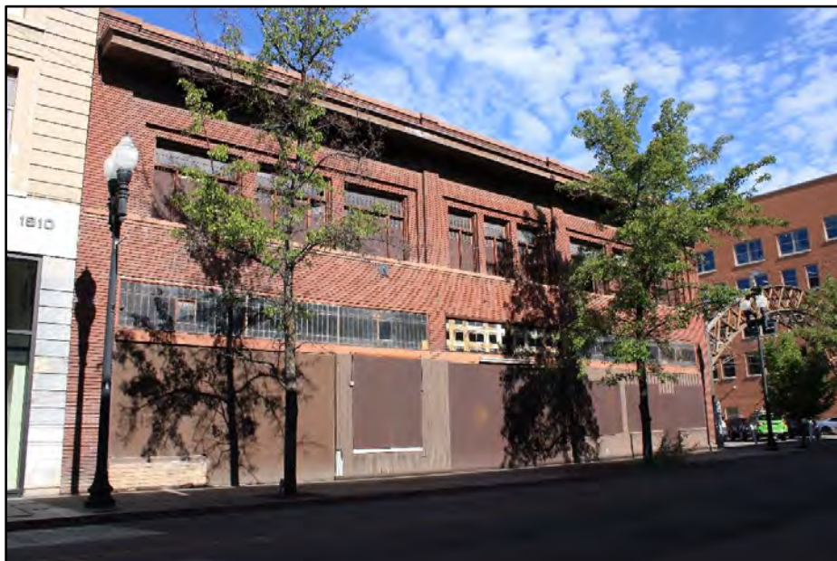
Photo 3. Hurst Building, 2439 Kiesel Avenue.
