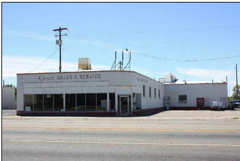
Photo 15. Kiesel Sales and Service, 3190 Washington Boulevard.
