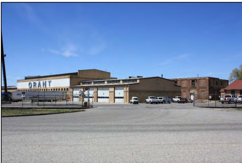
Photo 31. California Packing Company (warehouse), 910 W 24th Street, at the southwest corner of West 24th Street and Pennsylvania Avenue.
