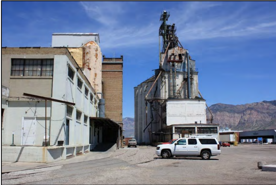
Photo 26. Sperry Flour Company (Royal Plant), 206 W 29th Street, at the northwest corner of 29th Street and Reeves Avenue.
