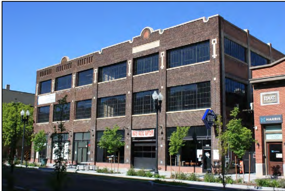
Photo 8. Thorstensen Building, 2331-2337 Grant Avenue.
