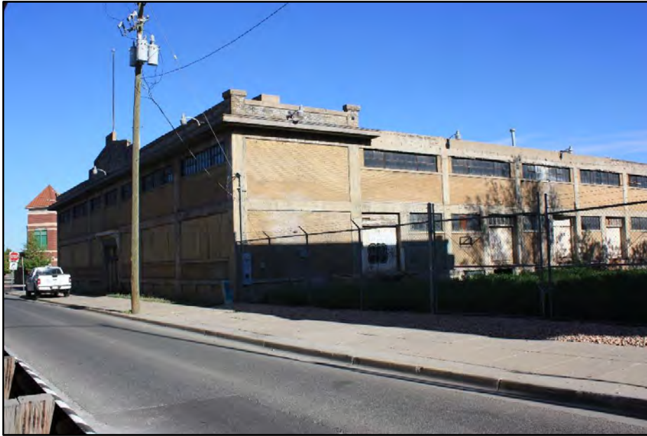
Photo 10. Interstate Terminal Warehouse, 2386 Wall Avenue, aka 118 24th Street.
