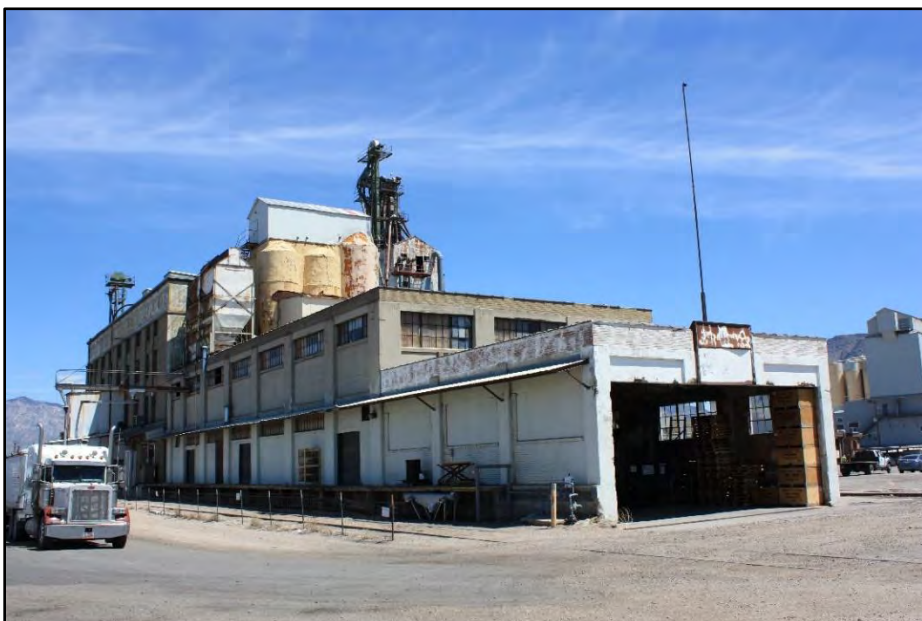
Photo 27. Sperry Flour Company (Royal Plant), 260 W 29th Street, at the northwest corner of 29th Street and Reeves Avenue.
