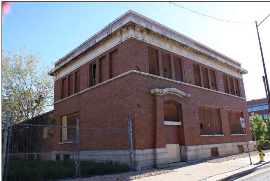
Photo 23. Denver & Rio Grande Railroad Company Freight Office and Warehouse, 128–132 24th Street.
