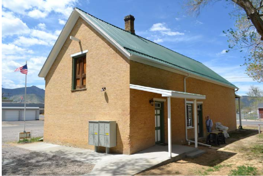
Photo 3 of 20: East and north elevations. Camera facing southwest.
