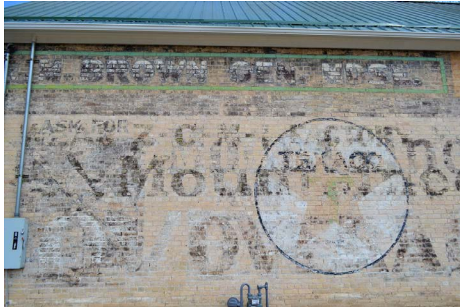
Photo 7 of 20: Detail of south elevation ghost signs. Camera facing north.
