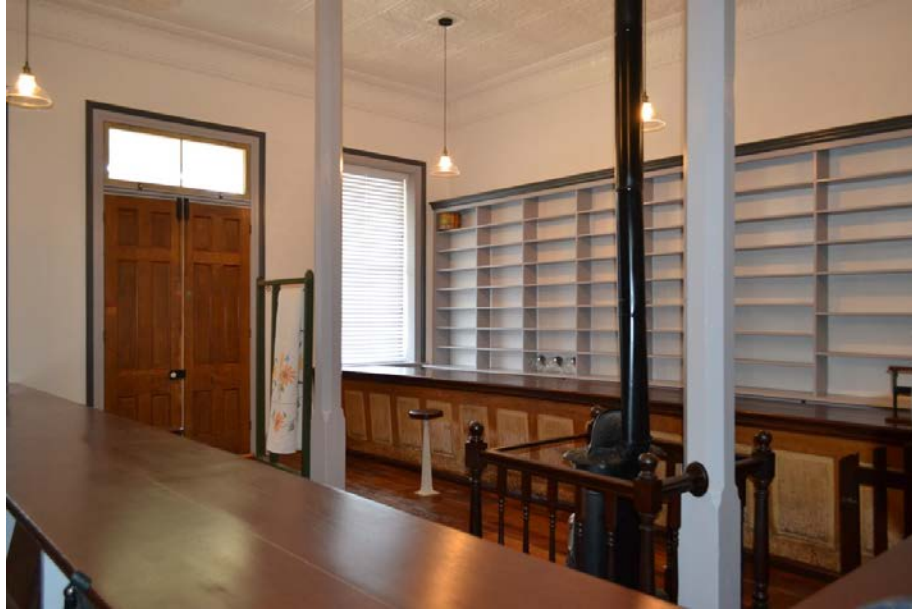
Photo 9 of 20: Interior of retail space. Camera facing northwest.
