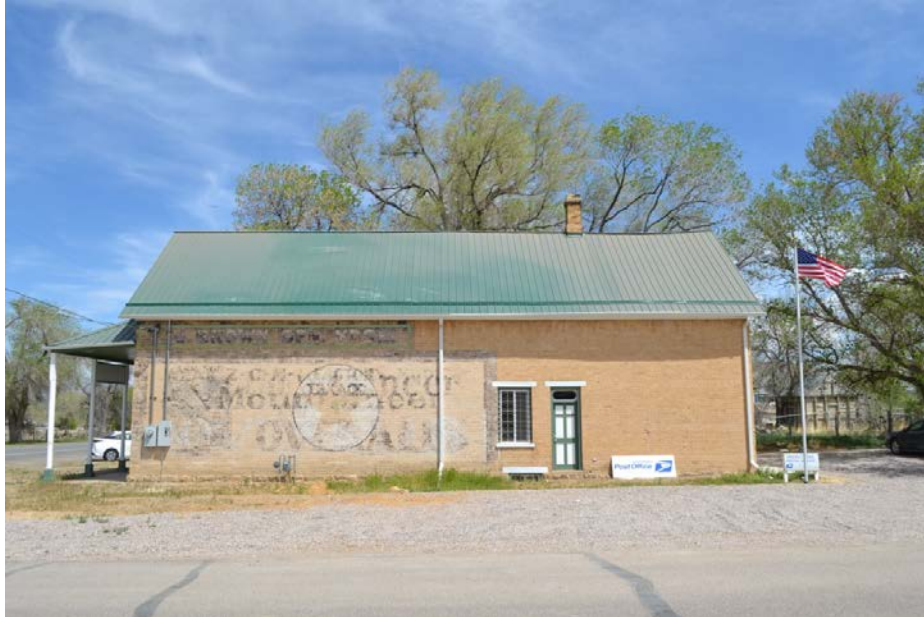
Photo 5 of 20: South elevation. Camera facing north.
