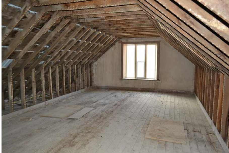
Photo 19 of 20: Upper level living space. Camera facing southwest.
