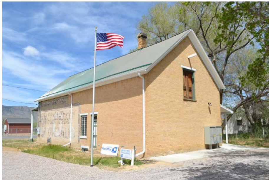
Photo 4 of 20: South and east elevations. Camera facing northwest.
