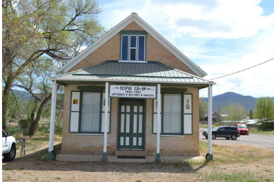
Photo 1 of 20: View of the West (front) elevation. Camera facing east.
