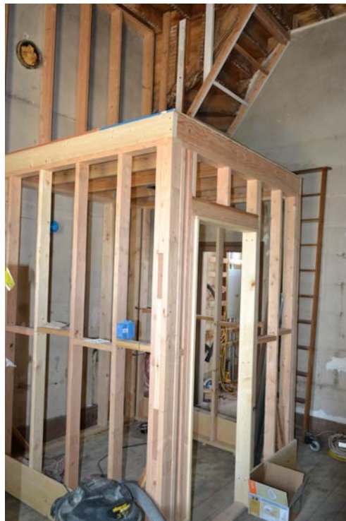
Photo 12 of 20: Interior of storage space—restroom construction . Camera facing southeast.
