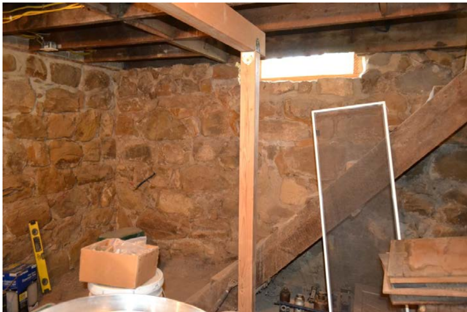
Photo 16 of 20: Interior of cellar space. Camera facing southeast.
