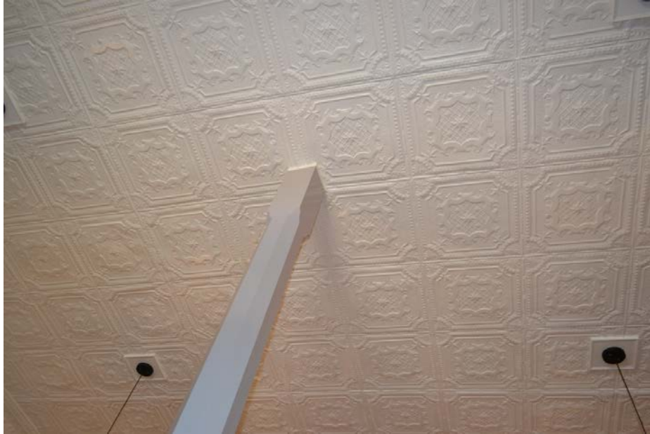
Photo 11 of 20: Interior of retail space—tin roof detail. Camera facing up
