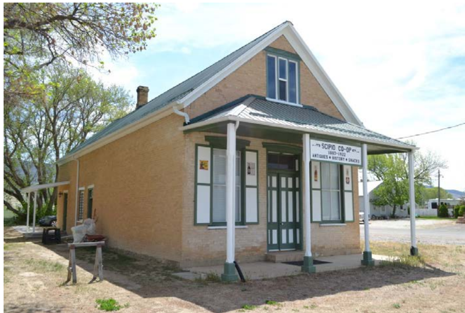
Photo 2 of 20: View of the north and west (back) elevations. Camera facing southeast.
