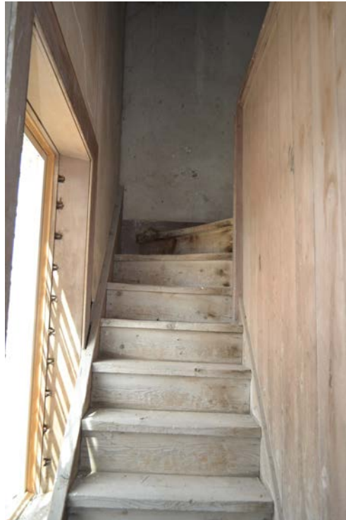
Photo 17 of 20: Interior staircase detail. Camera facing west.
