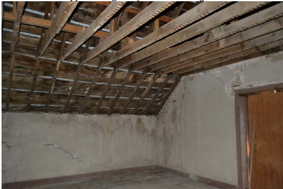
Photo 18 of 20: Interior of upper level granary. Camera facing northeast.
