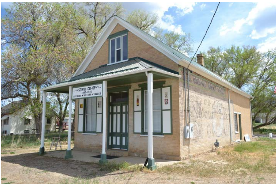
Photo 6 of 20: South and west elevations. Camera facing northeast.
