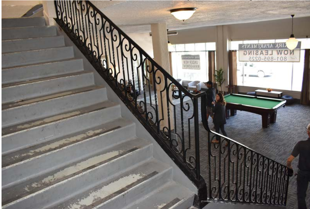
11 of 42: Stair detail looking into the hotel lobby. Camera facing northwest.
