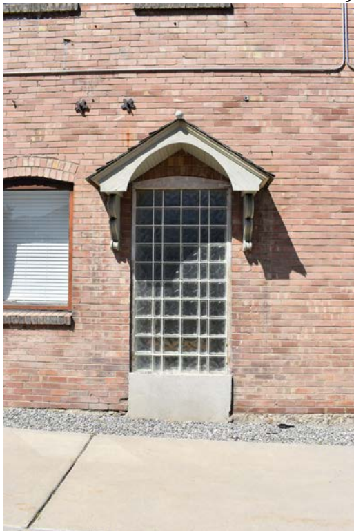
10 of 42: Fenestration detail on east façade of hotel. Camera facing west.
