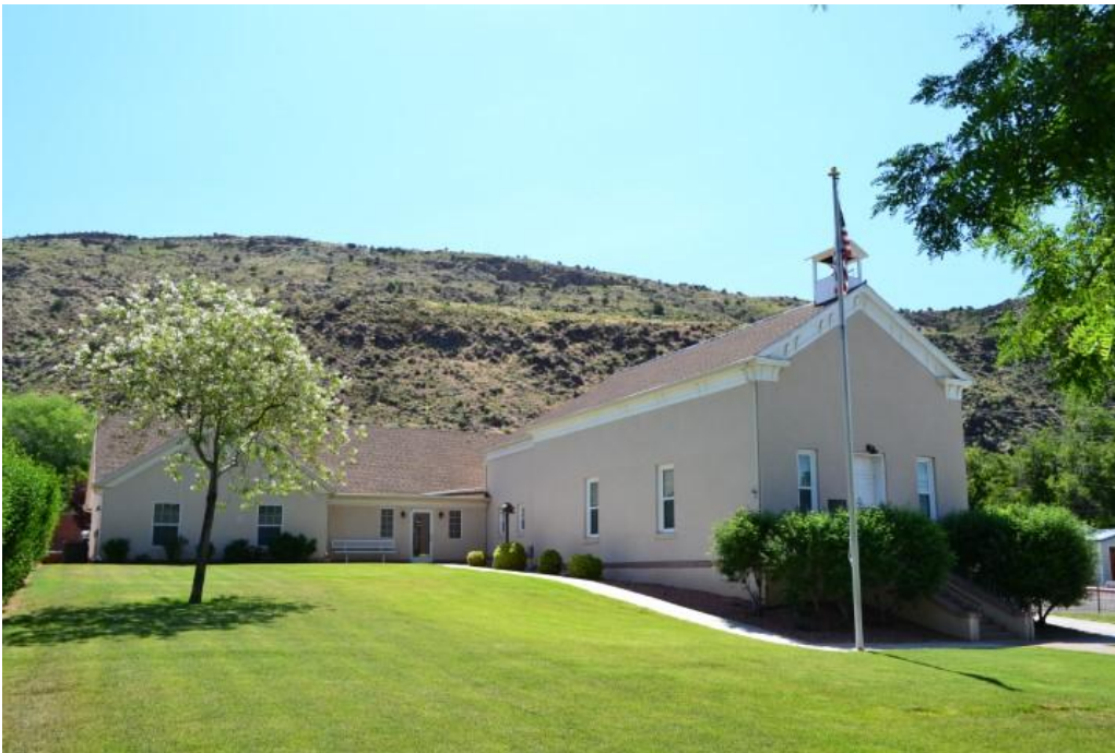
Photograph 2 of 20 West and north elevations. Camera facing southeast.
