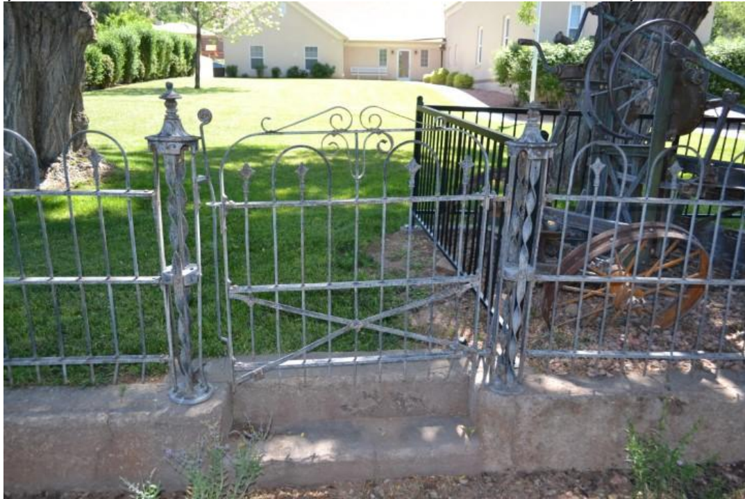
Photograph 17 of 20 Iron fence/gate detail. Camera facing east.
