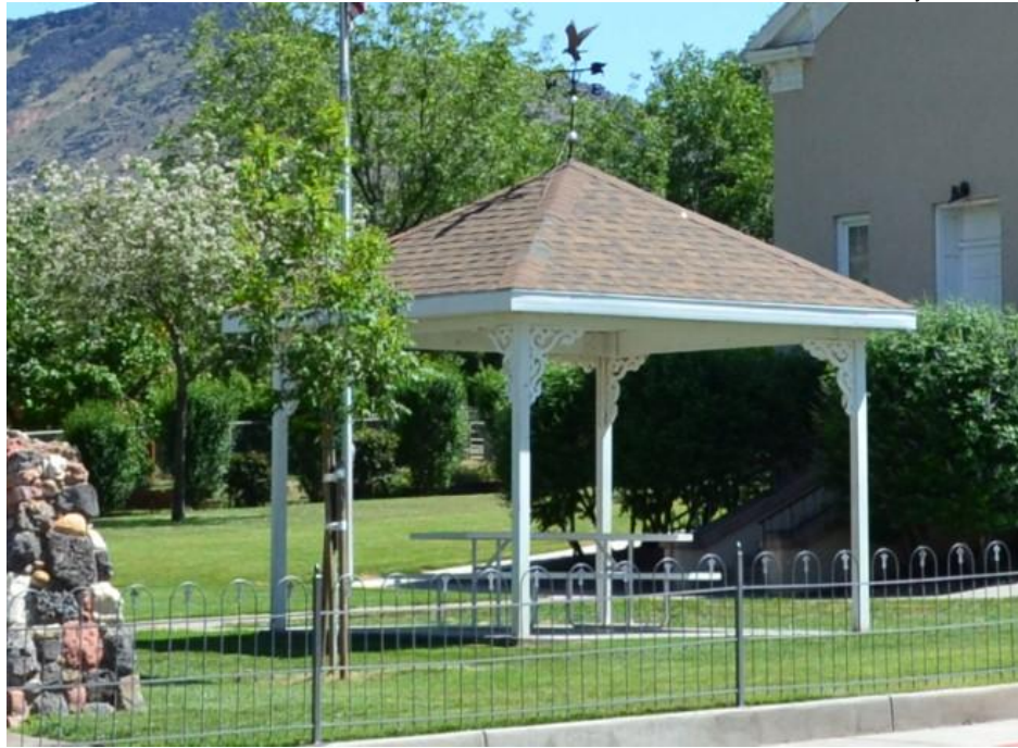
Photograph 19 of 20 Canopy/picnic structure. Camera facing northeast.
