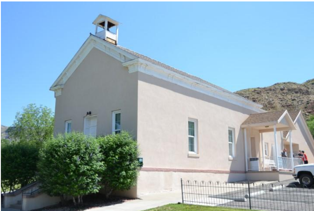
Photograph 8 of 20 West and south elevations. Camera facing northeast.
