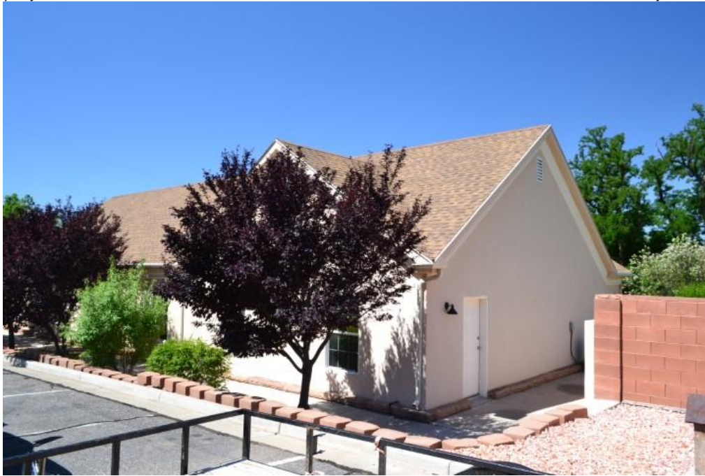
Photograph 5 of 20 East and north elevations of addition. Camera facing southwest.
