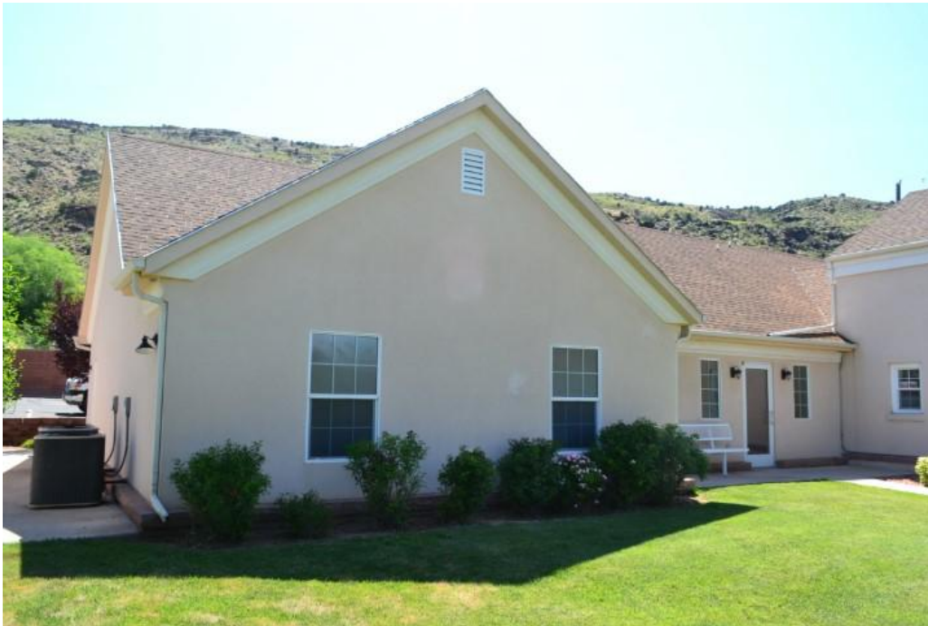
Photograph 4 of 20 West and north elevations of addition. Camera facing southeast.
