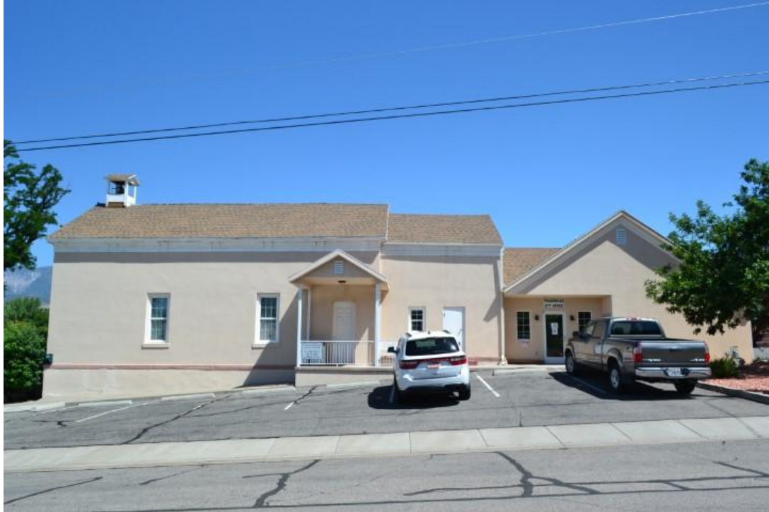
Photograph 7 of 20 South elevation. Camera facing north.
