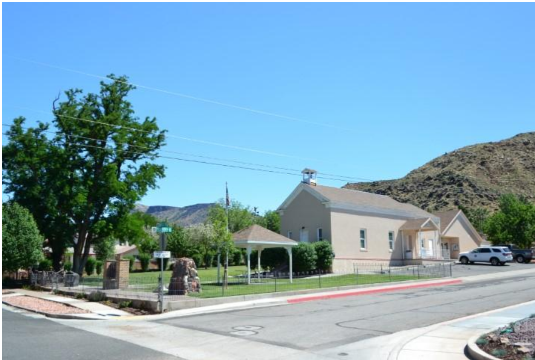
Photograph 14 of 20 Overview of property. Camera facing northeast.
