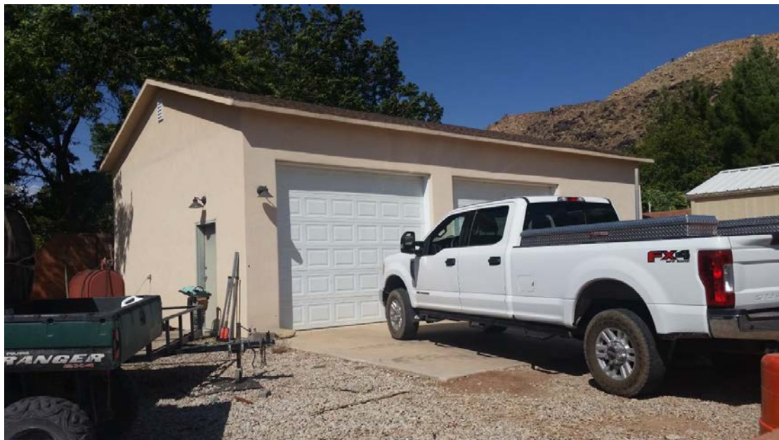
Photograph 20 of 20 Garage (left) & metal shed (far right). Camera facing northeast. (Photo, June Jeffery, September 2019)
