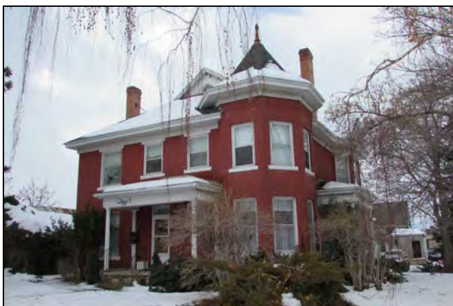
Figure 1. Clegg House; looking southwest
