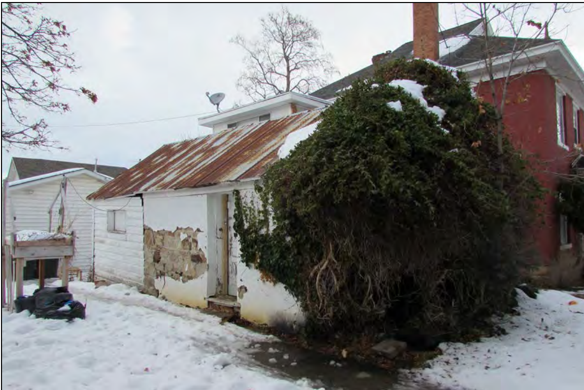
17 of 18. Clegg House—contributing cold storage/workshop; camera facing west-northwest
