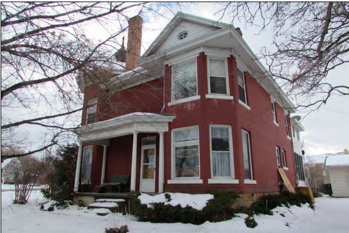
4 of 18. Clegg House—north and west elevations; camera facing south-southeast
