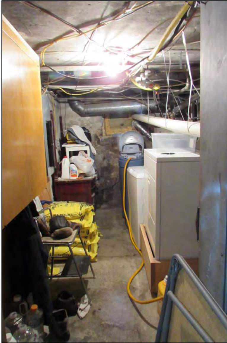
8 of 18. Clegg House—basement; view to the west
