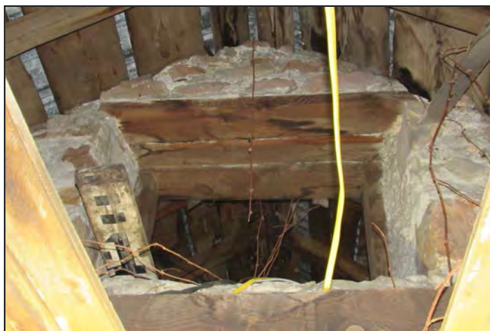
Figure 5. Attic opening in cold storage/workshop; looking west
