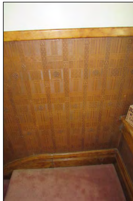
Figure 3. Wallpaper in stairwell
