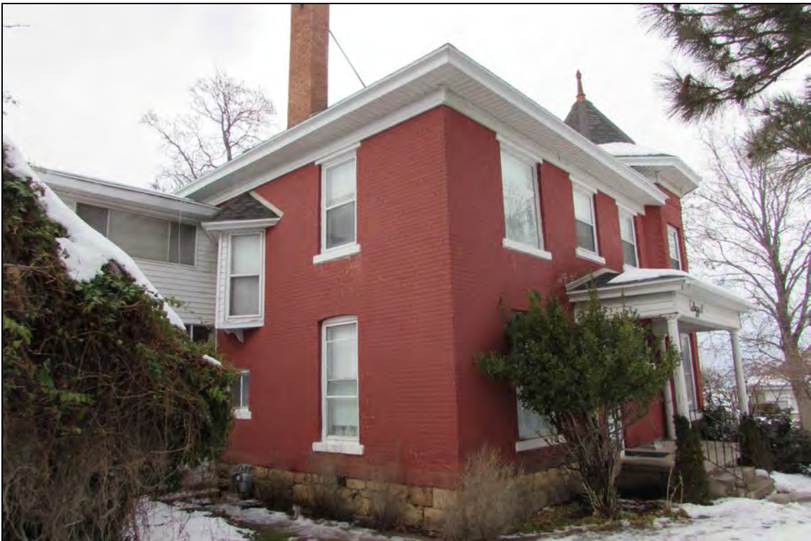
6 of 18. Clegg House—south and east elevations; camera facing northwest
