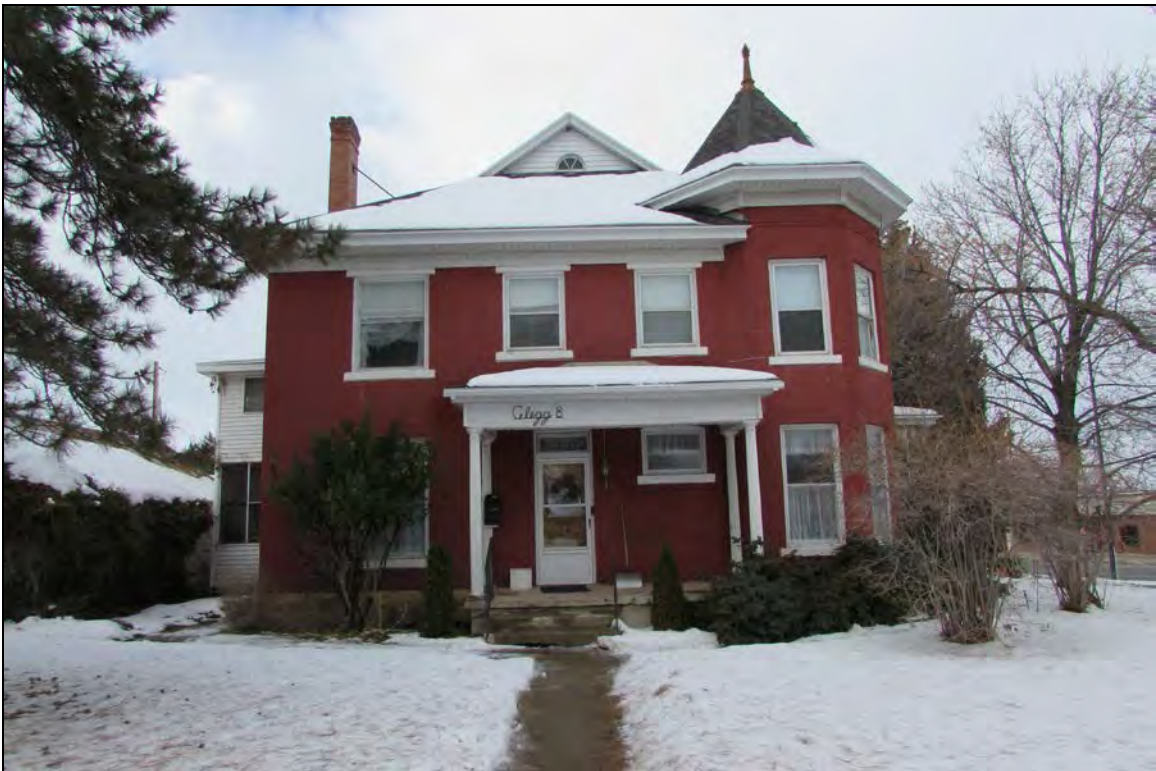
2 of 18. Clegg House—east elevation; camera facing west
