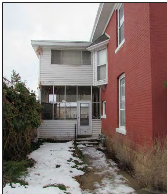
Figure 2. Clegg House addition; looking west
