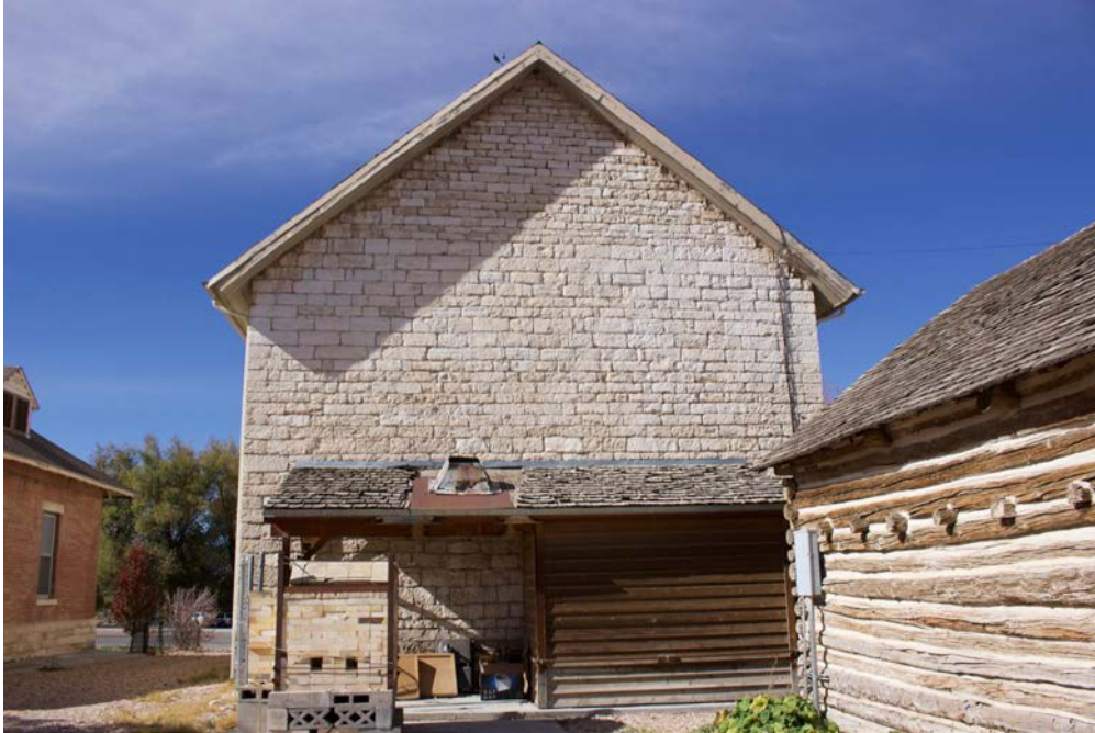
5 of 21: East elevation of granary. Camera facing west. (Photo by Jamyn Maddox, 10/31/18)
