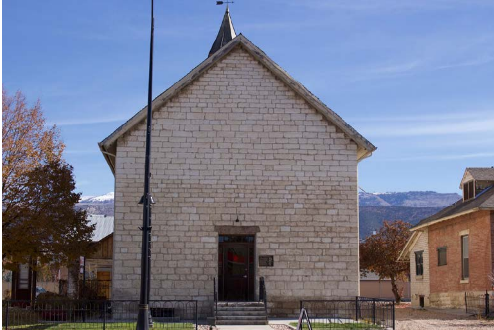
1 of 21: West elevation of granary. Camera facing east. (Photo by Jamyn Maddox, 10/31/18)
