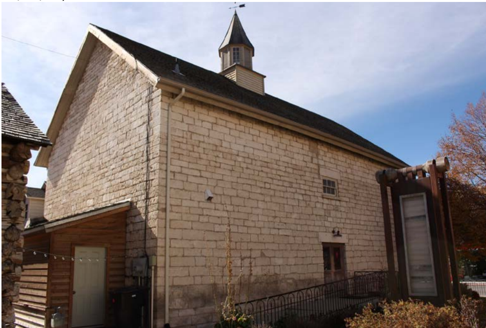
6 of 21: North-east corner of granary. Camera facing south-west. (Photo by Jamyn Maddox, 10/31/18)
