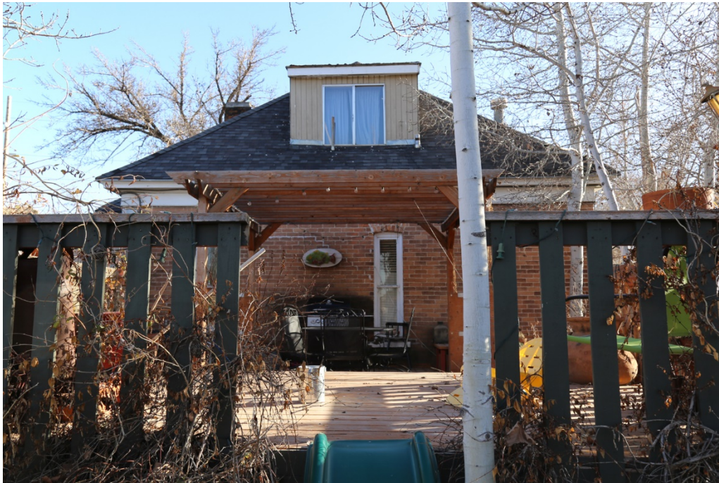
Photograph 5 North elevation of house. Camera facing south.
