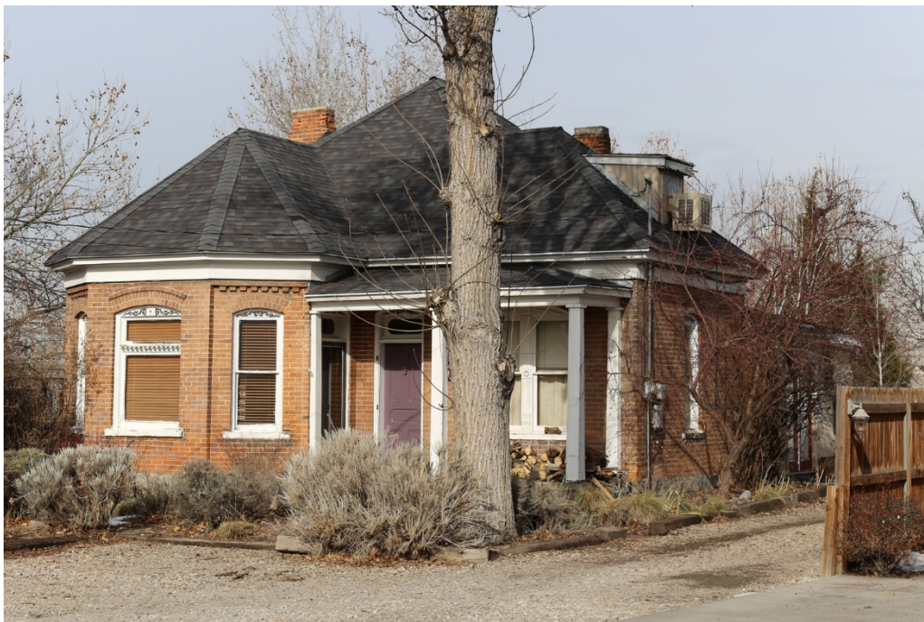
Photograph 2 South and east elevations of house. Camera facing northwest.
