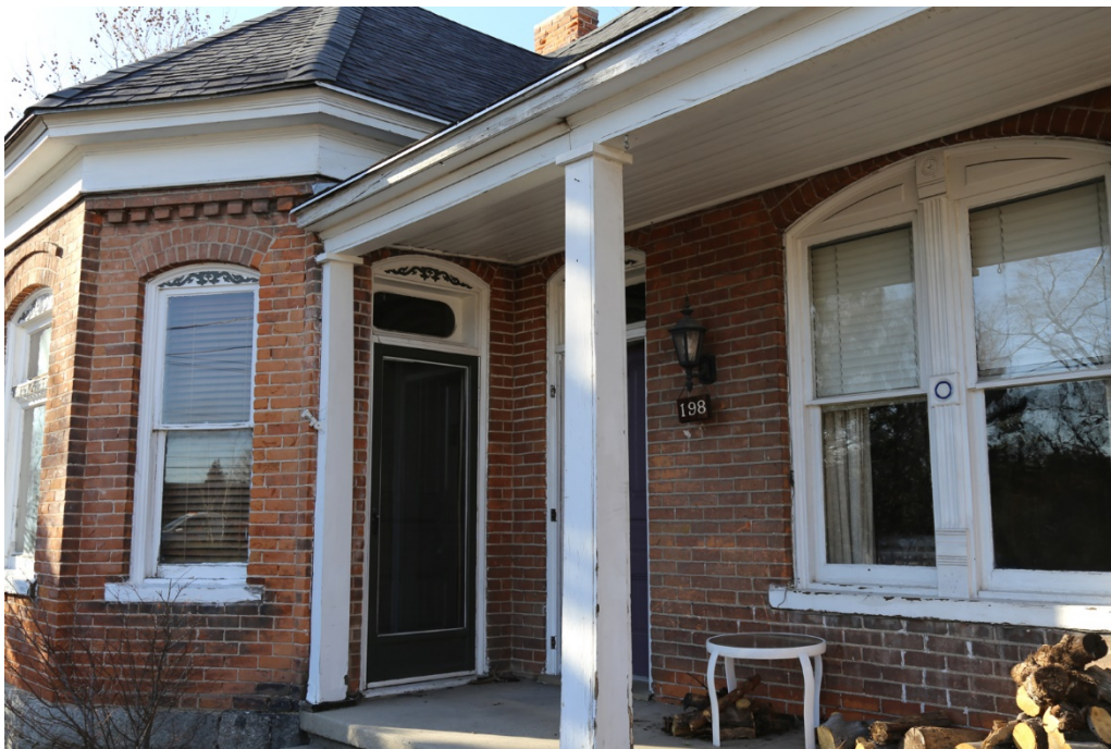
Photograph 6 South elevation of house, porch details. Camera facing northwest.
