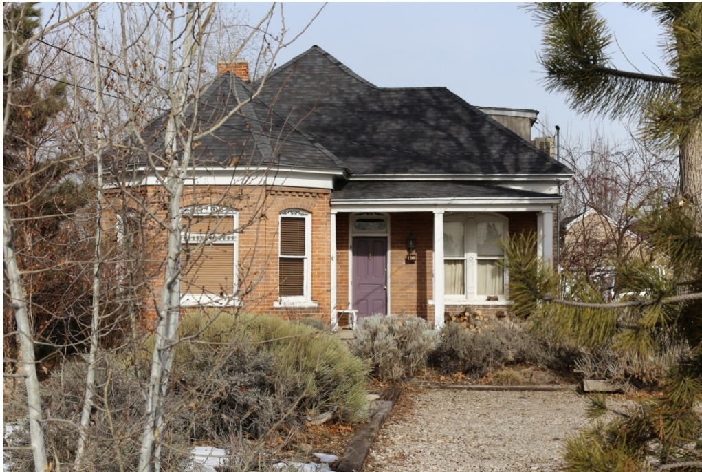
Photograph 1 South elevation of house, view of site with garage on right. Camera facing north.
