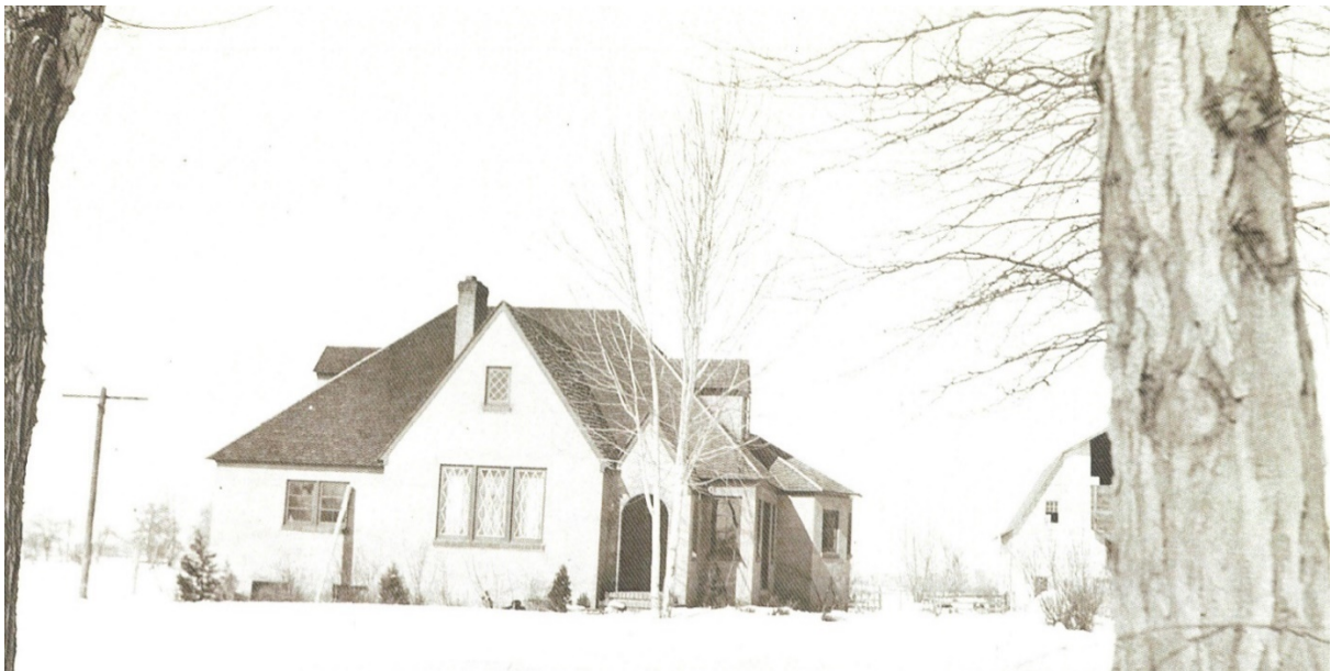
FIGURE 1 Smith House, circa 1958 South elevation. Camera facing north. Photograph courtesy Salt Lake County Archives, Tax Assessor's Photograph.
