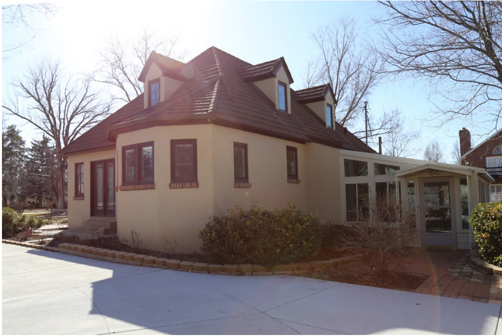
Photograph 3 East and north elevations of house. Camera facing southwest.
