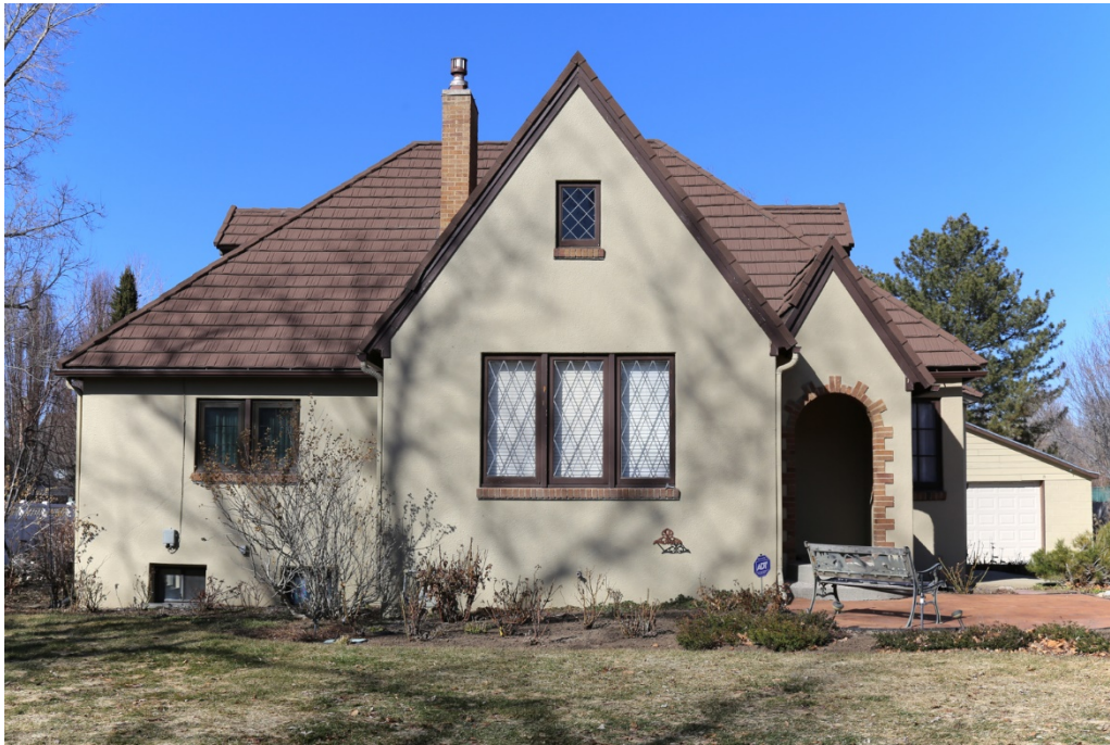
Photograph 1 South elevation of house, view of site with garage on right. Camera facing north.
