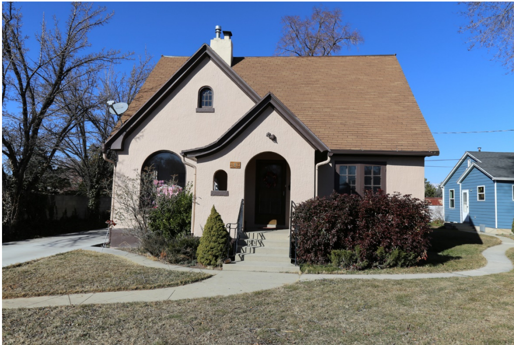
Photograph 1 South elevation of house, view of site with adjacent house on right. Camera facing north.
