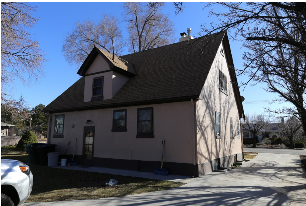
Photograph 4 North and west elevations of house. Camera facing southeast.
