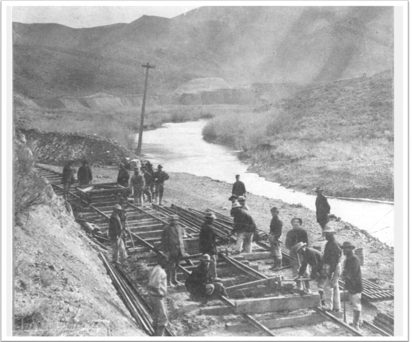
Photo: Railroad workers curving iron rails, 12-Mile Canyon, Nevada, 1868
