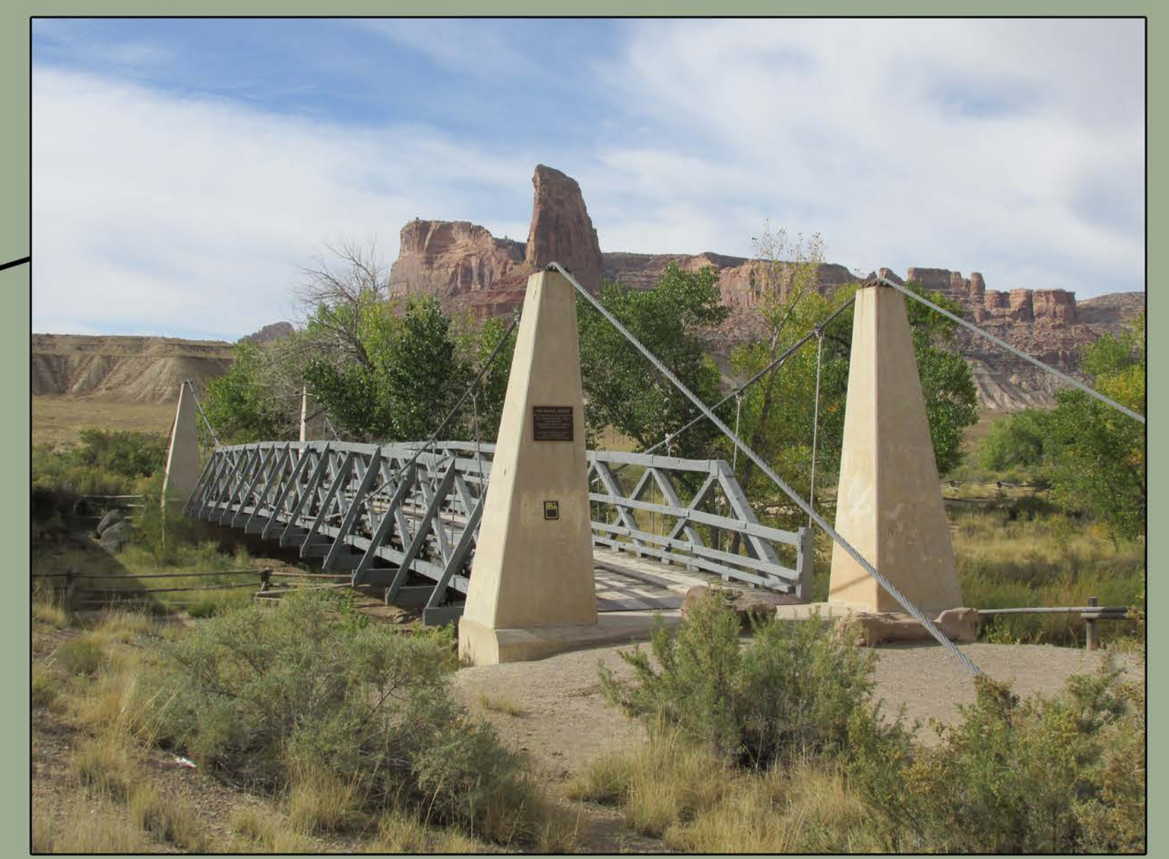
Buckhorn Wash Bridge, Emery County, built in 1936.
