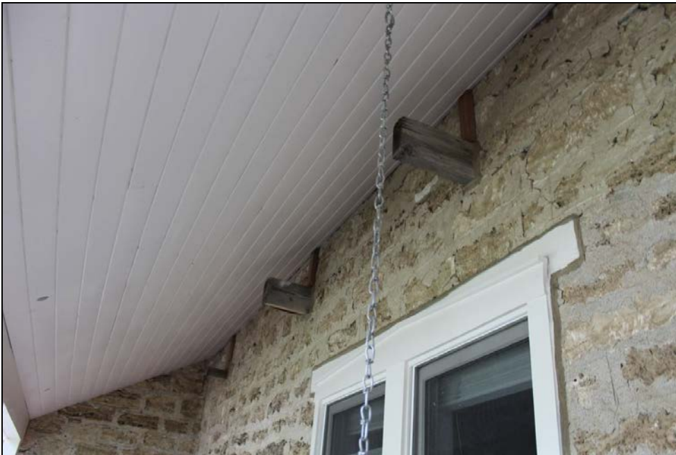
10 of 16. Detail of beams extending from west elevation under modern porch. Camera facing northwest.
