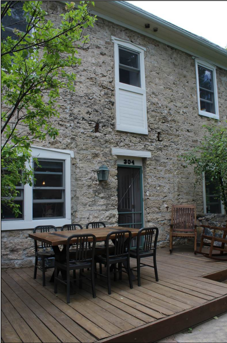
7 of 16. North elevation. Camera facing southwest. Note infilled door opening on second story and beams where a porch may have been attached.
