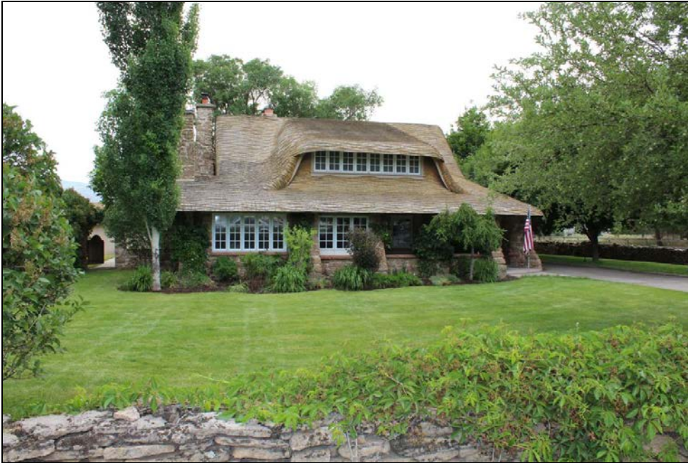
1 of 36. West elevation. Camera facing east.
