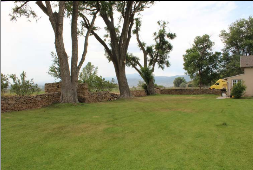
31 of 36. Structure 1 (stone wall) on south and east sides of property. Camera facing south.
