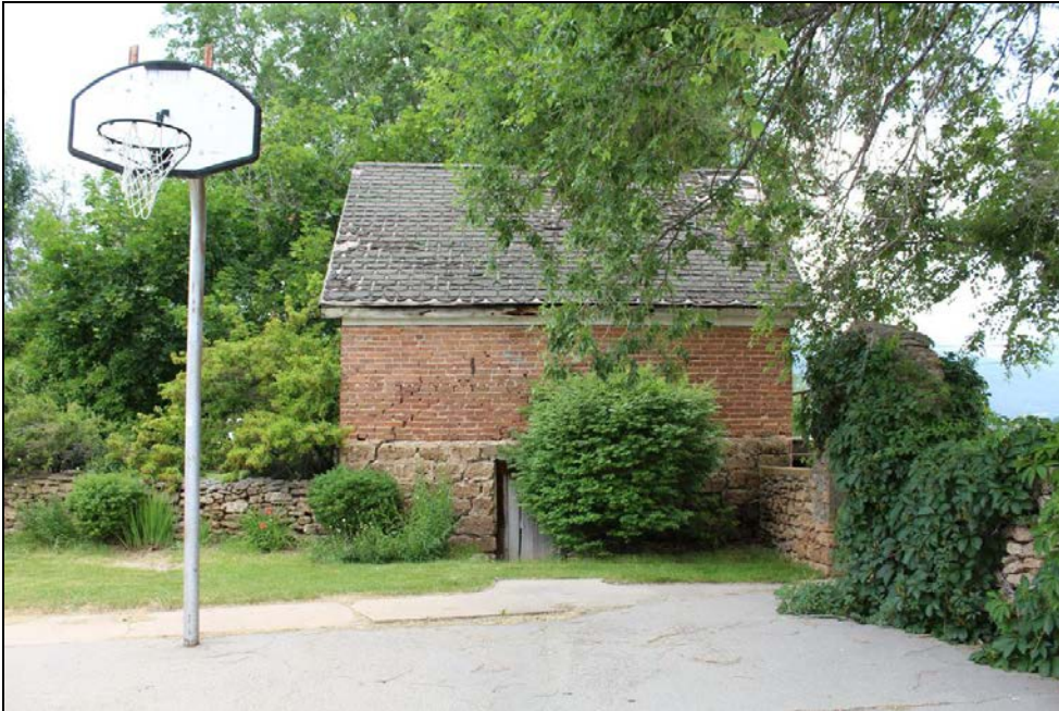
23 of 36. Outbuilding (creamery/granary). Camera facing west.
