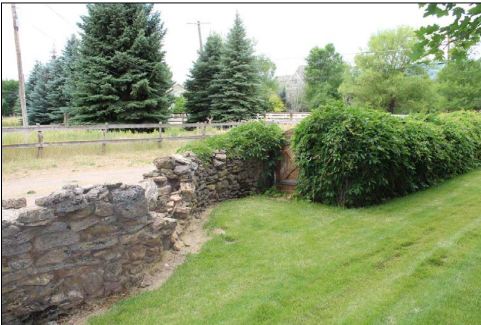
32 of 36. Structure 1 (stone wall) on south side of property. Camera facing southwest.
