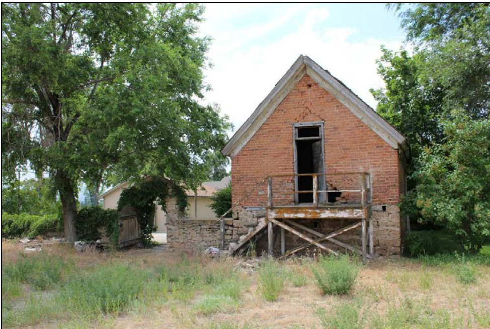
20 of 36. Outbuilding 1 (creamery/granary). Camera facing south.
