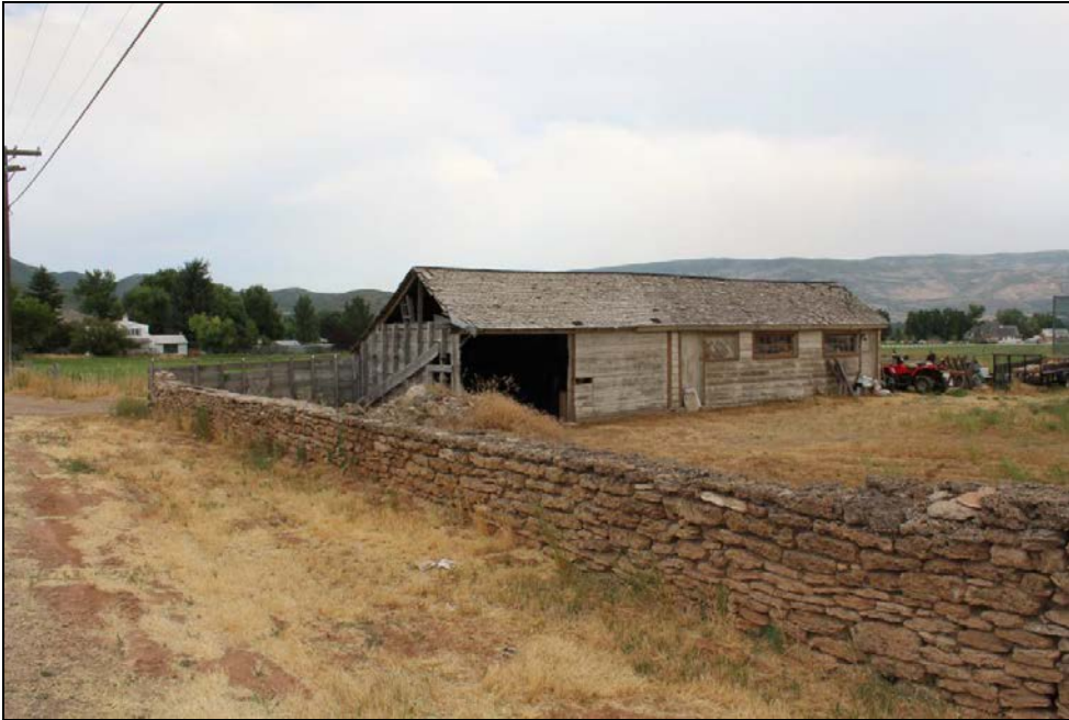
33 of 36. Structure 1 (stone wall). Camera facing northwest. Note Outbuilding 3 in the background.
