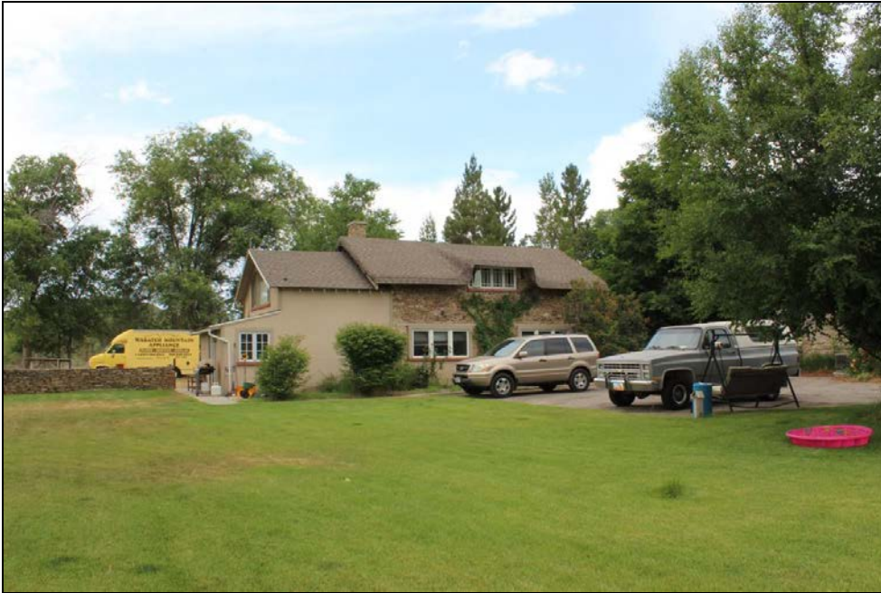
27 of 36. Outbuilding 3 (original garage). Camera facing south.
