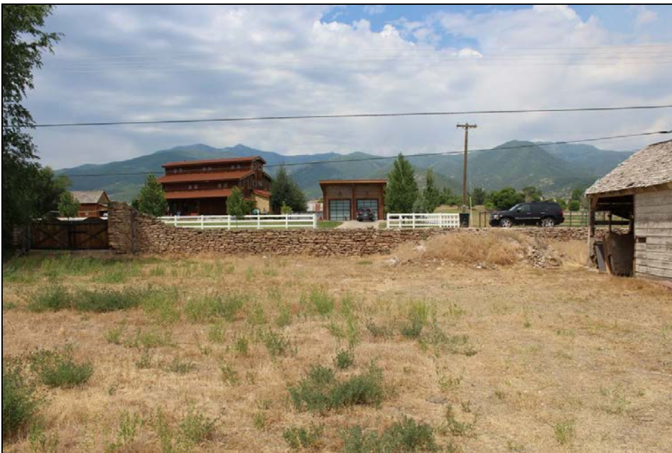
26 of 36. Outbuilding 2 (horse barn and shed). Camera facing west. Note missing section of building to the south of the remaining building
