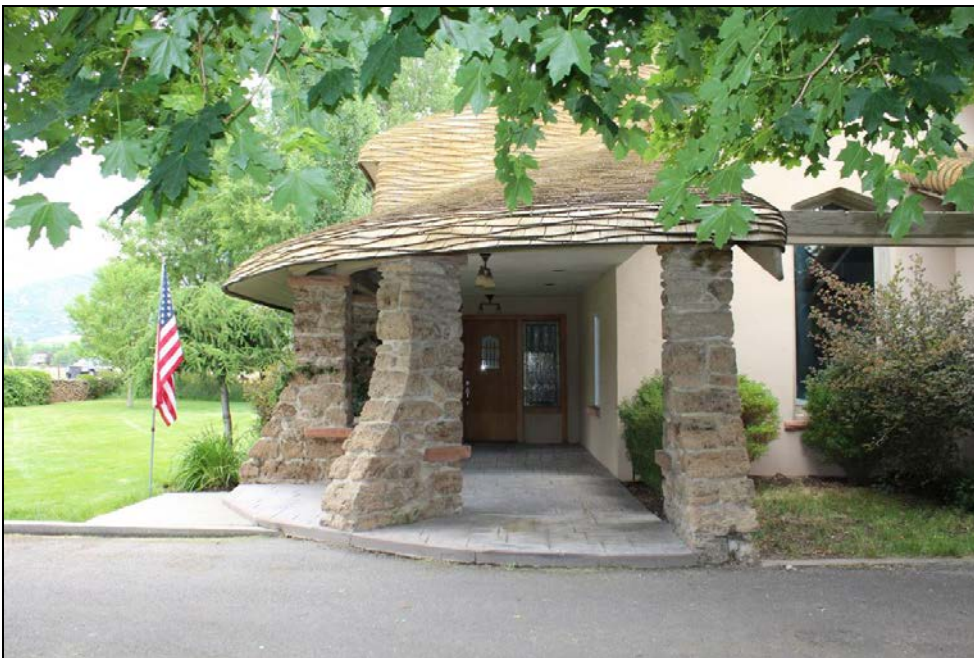
4 of 36. South elevation. Camera facing north.
