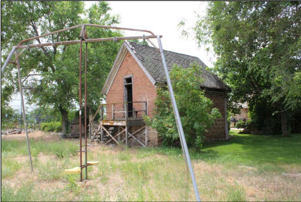
21 of 36. Outbuilding 1 (creamery/granary). Camera facing southeast.
