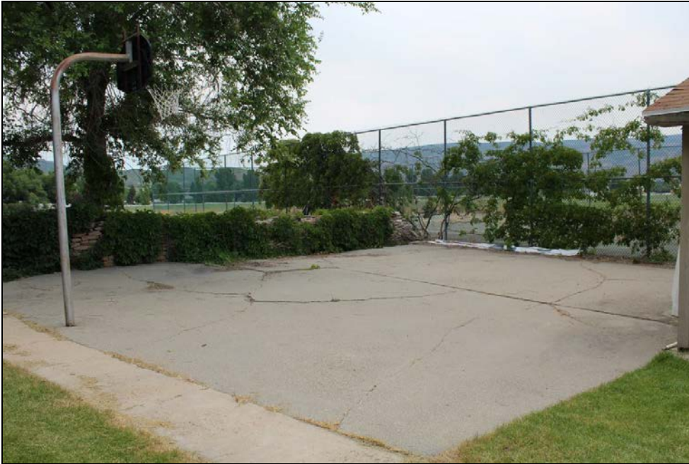
35 of 36. Structure 2 (basketball court). Camera facing northeast.
