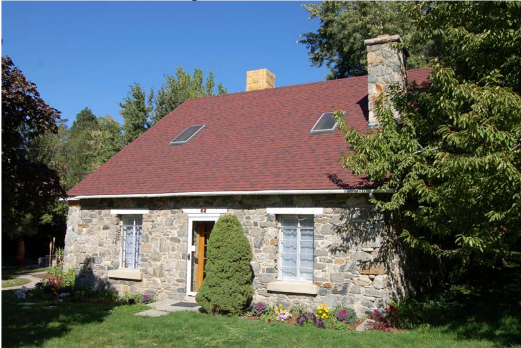
Photograph 7. 82 West 600 North. Camera facing north.
