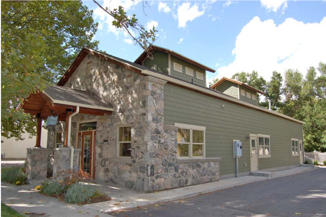
Photograph 24. 63 North Main Street. Camera facing southwest.
