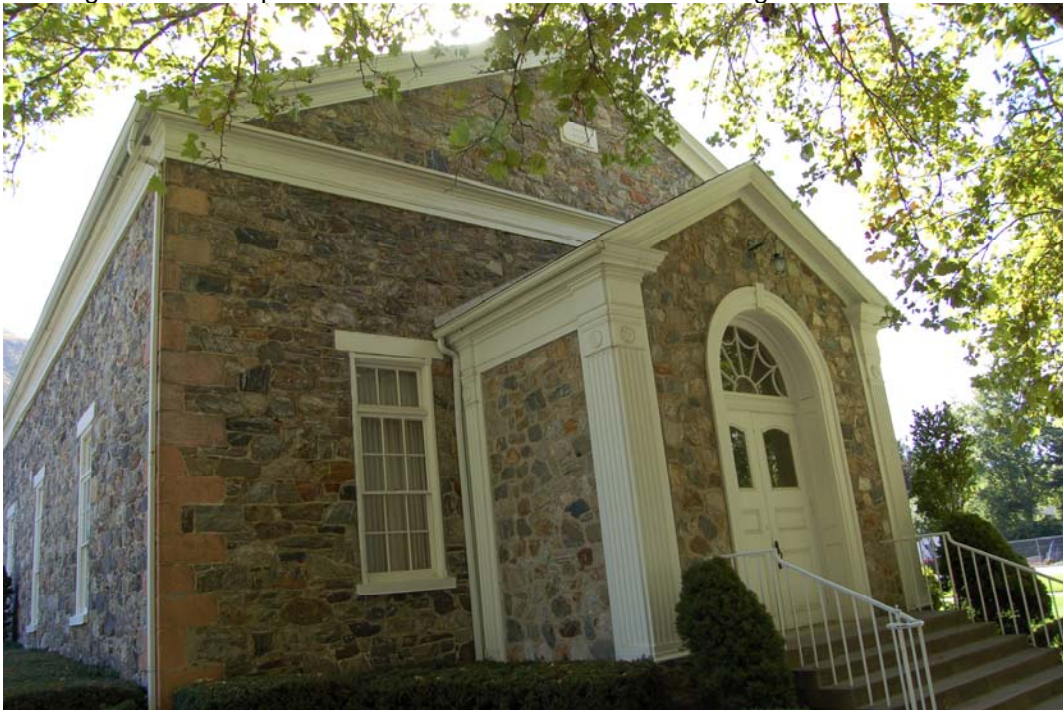
Photograph 11. Farmington Rock Chapel. 272 North Main Street. Camera facing southeast.
